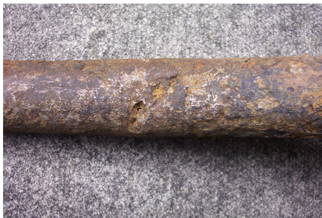
FIGURE 27.13 Pitting corrosion in an underground water pipe.
