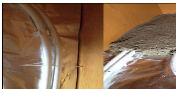
Fig. 6. Paraffin wax pipe installed in the floor.
