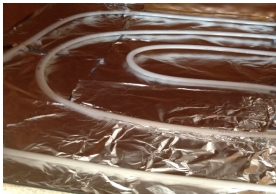
Fig. 2. Spiral water loop pipes installation.
