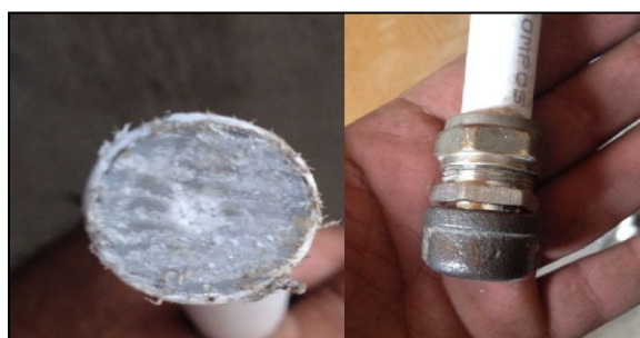
Fig. 5. Paraffin wax pipe installed in the floor
