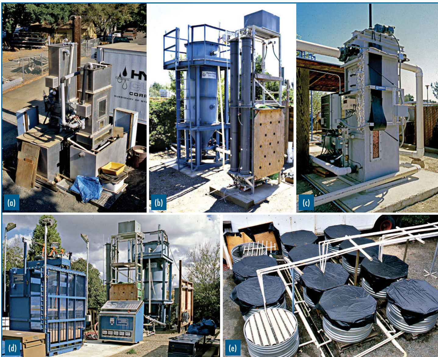
Filtration studies at the UCD campus WWTP:
