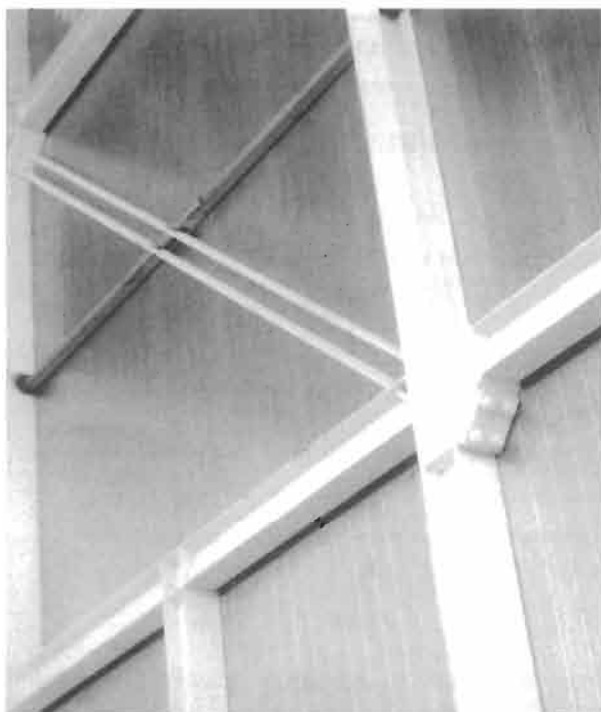
Fig. 1. Prestressed steel frame using two bars.
