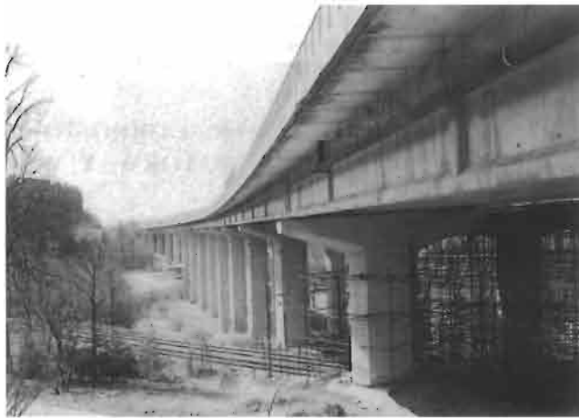
Fig. 1. Prestressed concrete construction of the viaduct.
