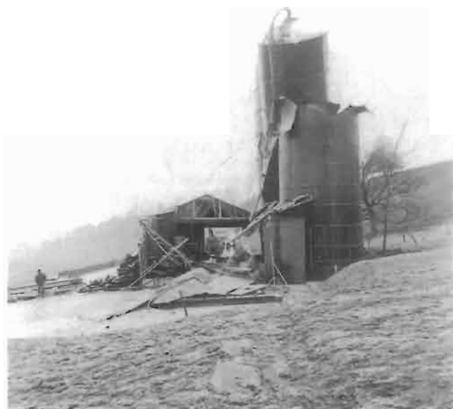
Fig. 1. Damaged silos: view of the site.
