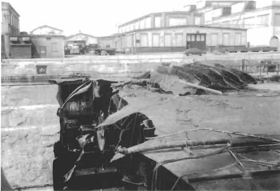
Fig. 12. View of the deck plate fracture: part of the deck and longitudinal ripped out during final fracture is also shown.
