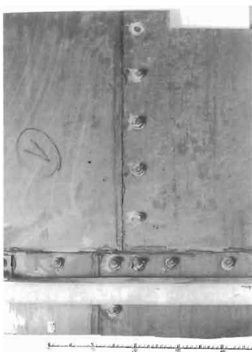
Fig. 2. Bolted joints of the sheets used for the silo. In the lower part, a reinforcement ring was attached.
