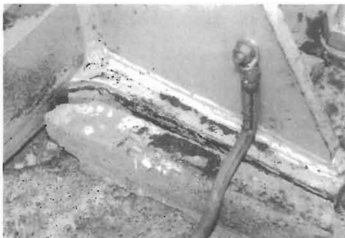
Fig. 7. Typical detail of gusset welds showing complete absence of “rat hole” at the junction of the three members.
