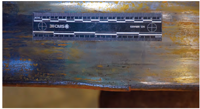
Fig. 65 Top view of damage to area 1 from Fig. 63
