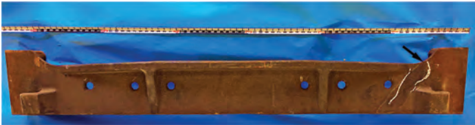
Fig. 113 Overall view of as-received beam. Crack location is indicated by chalk and arrow on right side of image
