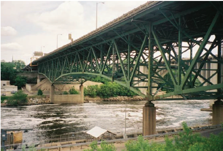
Figure 6-2. Center span of the I-35W Bridge before collapse.
