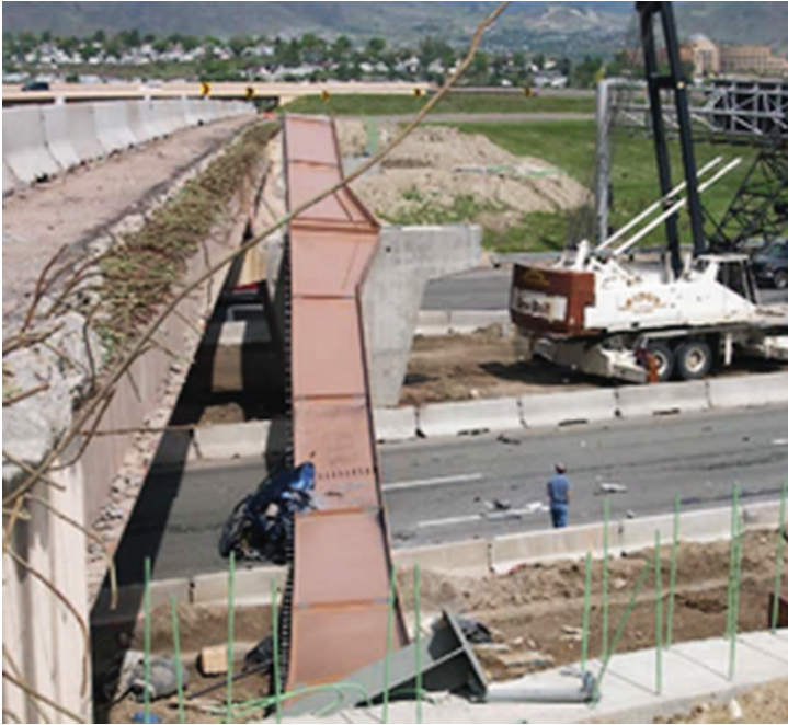
Figure 4-1. Fallen girder and top portion of the accident vehicle on I-70 (looking north).
