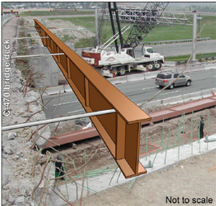
Figure 4-3. Diagram overlaid on photograph to show the girder that failed in its erected position along with the five braces in relation to the C-470 bridge deck.
