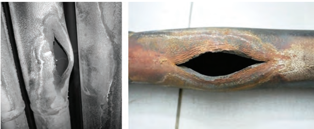
Fig. 6.36 Close-up views of a superheater tube at the failure location
