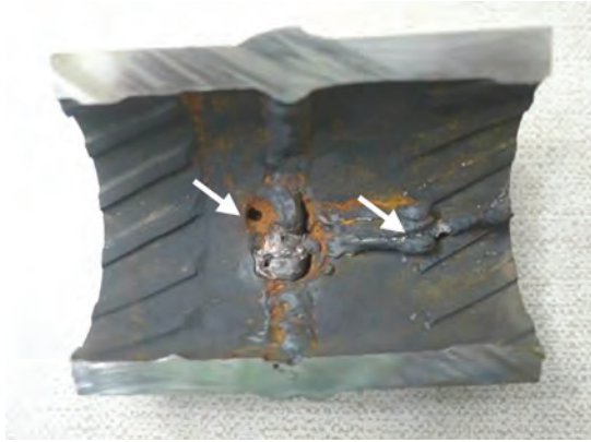
Fig. 6.163 Close-up view of ID surfaces showing puncture located at fusion zone of the butt weld. Uneven weld penetration forming nonuniform ridges at the weld line are shown. The weld metal had excess penetration (as shown by arrow).
