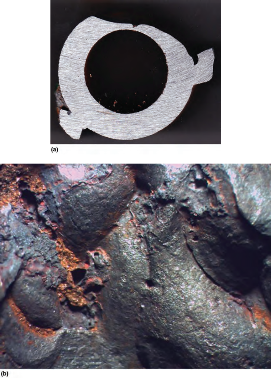
Fig. 6.168 (a) Transverse cross section of a tube at a few millimeters distance from the leak indicating metal wastage on outer surface. (b) Poor quality of welding with porosities and deep ripples, 6×
