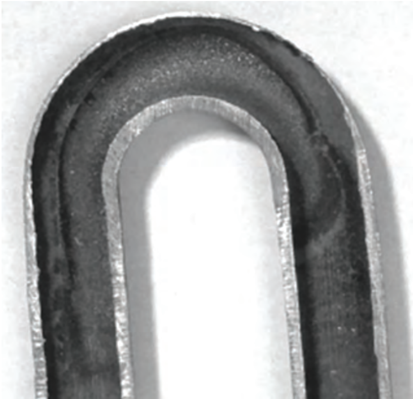
Fig. 6.80 Erosion-corrosion damage of economizer tube bend
