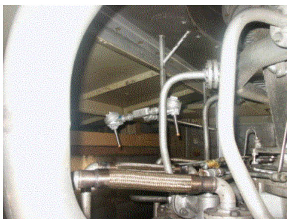
Figure 5.4: Heat detection in enclosure
