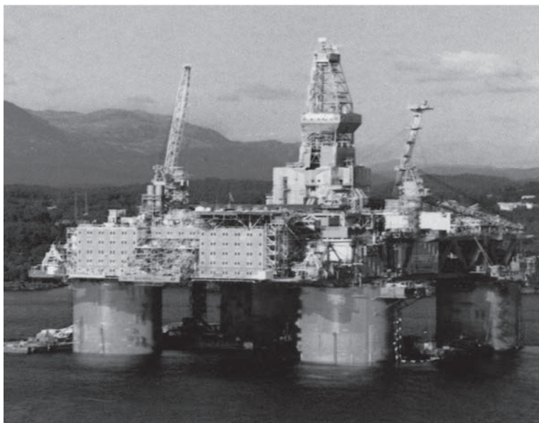
Fig. 3.1 Offshore oil rig with aluminum superstructure. Source: Ref 3.4–3.6, 3.11
