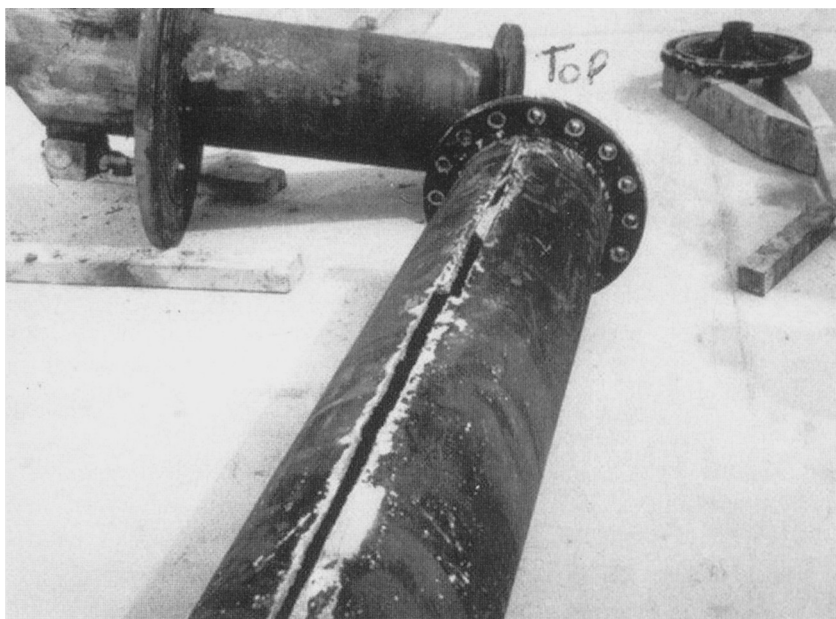
FIGURE 18.1 Corrosion of the beta phase in an NAB seam-welded pipe that had not been postweld heat treated. (Photograph courtesy of the Nickel Institute.) (See color section.)
