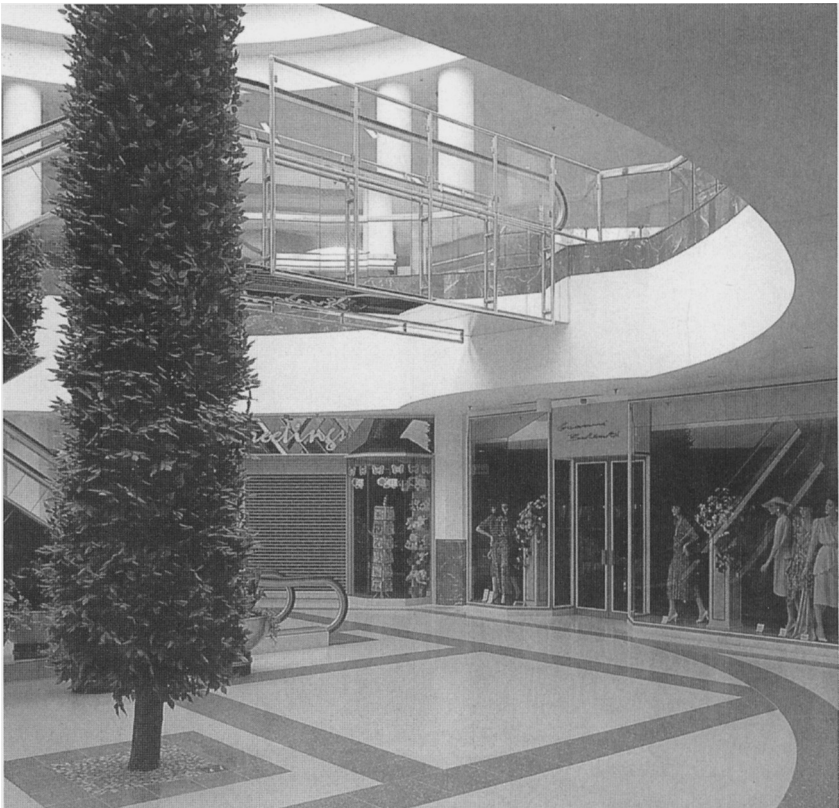
FIGURE 16.2 Brass escalator safety balustrades in a U.K. shopping center. (Photograph courtesy of the Copper Development Association.) (See color section.)
