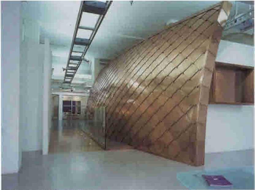
FIGURE 16.4 Copper used in a decorative internal curtain wall. (Photograph courtesy of NDM.)
