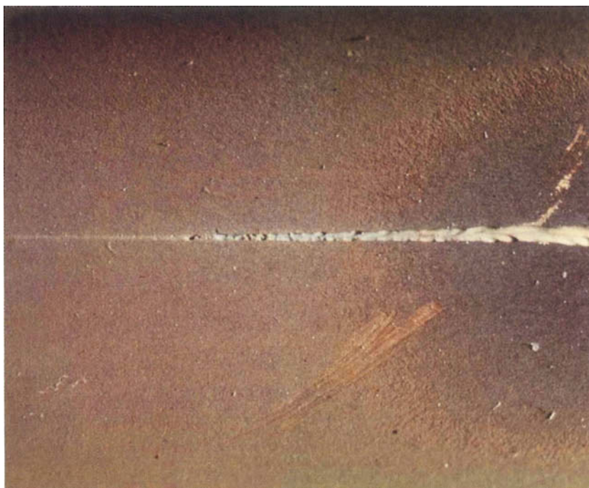
FIGURE 7.23 Erosion corrosion at a scratch line on an aluminum brass tube, where repassivation did not occur due to overchlorination.
