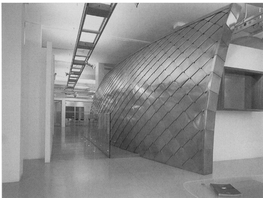
FIGURE 16.4 Copper used in a decorative internal curtain wall. (Photograph courtesy of NDM.) (See color section.)
