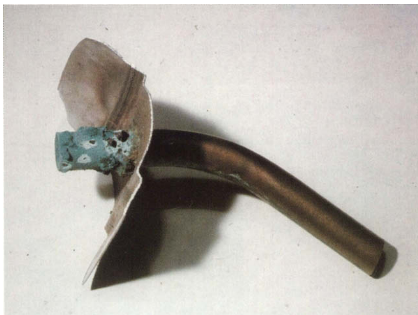
FIGURE 14.7 Severe corrosion of a copper pipe entering an SS hot water cylinder.
