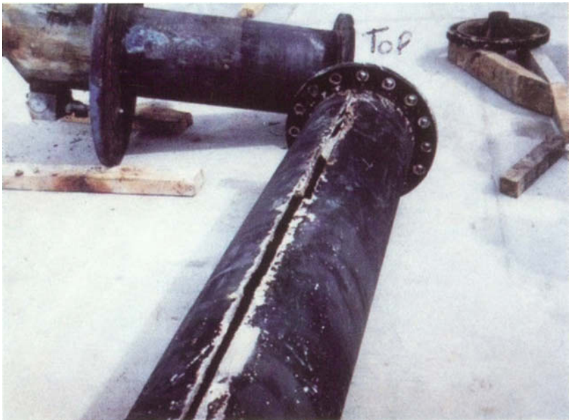
FIGURE 18.1 Corrosion of the beta phase in an NAB seam-welded pipe that had not been postweld heat treated. (Photograph courtesy of the Nickel Institute.)
