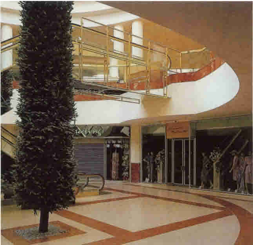
FIGURE 16.2 Brass escalator safety balustrades in a U.K. shopping center. (Photograph courtesy of the Copper Development Association.)
