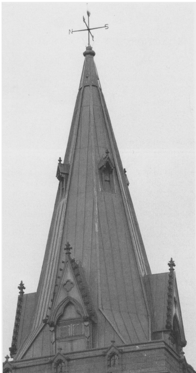
FIGURE 16.1 Copper-covered spire on St. Magnus Cathedral, Kirkwall, Scotland. (Photograph courtesy of the Copper Development Association.) (See color section.)
