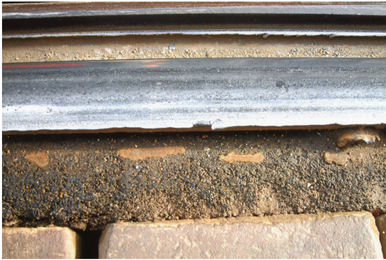
COLOR FIGURE 5.5 Cracking on a railroad track.
