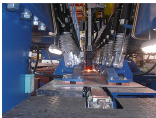
(b) Hybrid welding for floors
