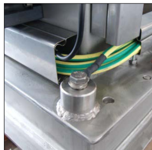
Picture 17 - Principle of earthing and bonding contact
