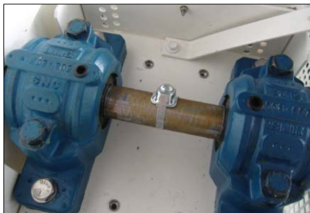
Pictures 13 and 14 - Principle of pulley and belt drive FAN proximity sensor – Inside and outside views
