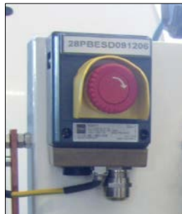
Picture 16 - Principle of FAN UNIT emergency push button
