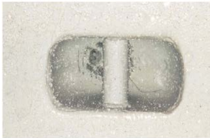
Recessed box tie down fitting
