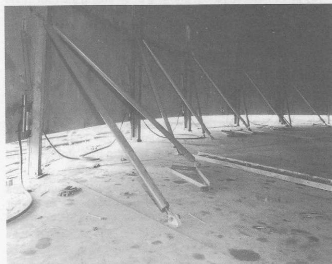
Figure 12.17 Arrangement of hydraulic climbing jacks Courtesy of McTay
