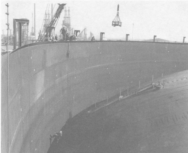
Figure 5.29 A 90 m diameter roof being air-lifted to the top of the tank
