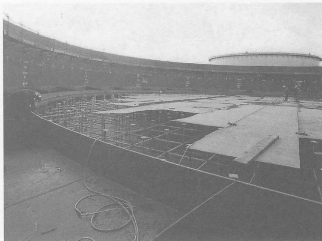
Figure 12.34 Scaffold support system for a single deck type roof of a 45 m diameter tank Courtesy of McTay
