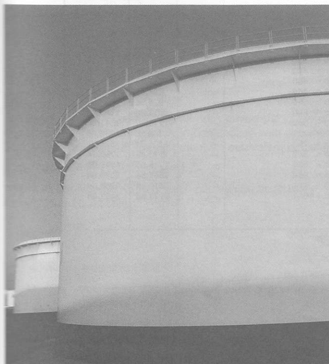
Figure 3.30 Primary wind girder
