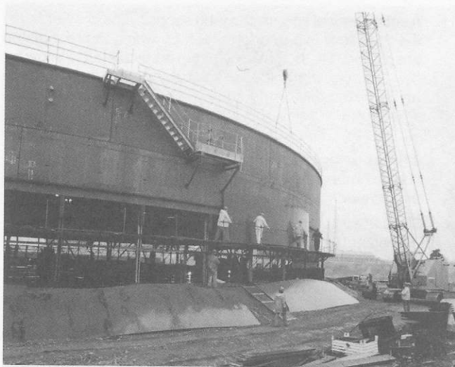
Figure 12.19 Tank being erected by the jacking method Courtesy of Whessoe
