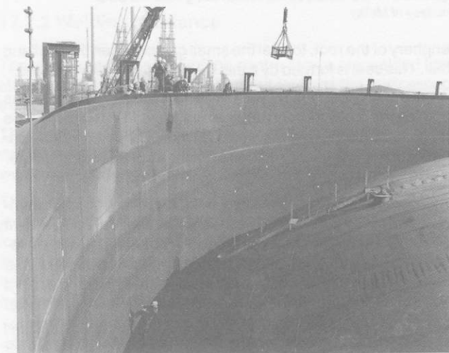
Figure 12.24 31 m diameter dome roof being air-lifted into place
