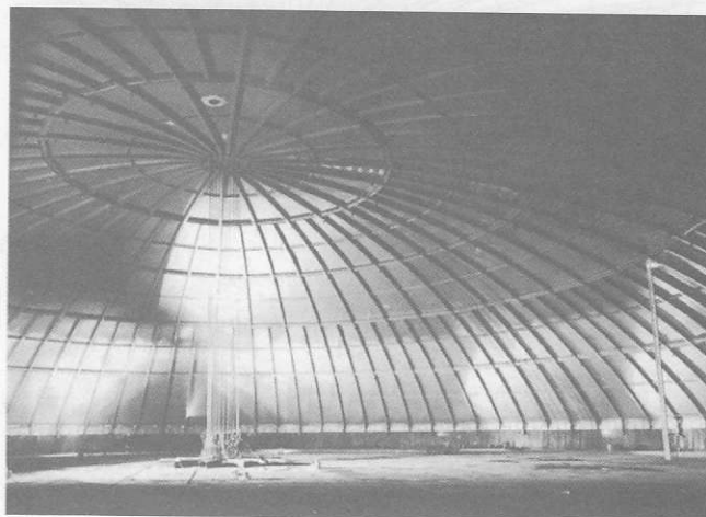
Figure 5.28 90 m diameter internally-framed dome roof completed and ready to be air-lifted (note the stabilisation cables attached to the centre of the floor)
