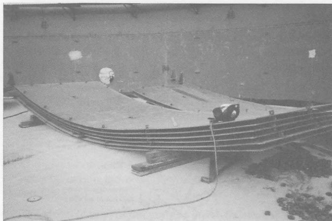
Figure 12.6 Welding of blank erection nuts to the shell plates Courtesy of McTay
