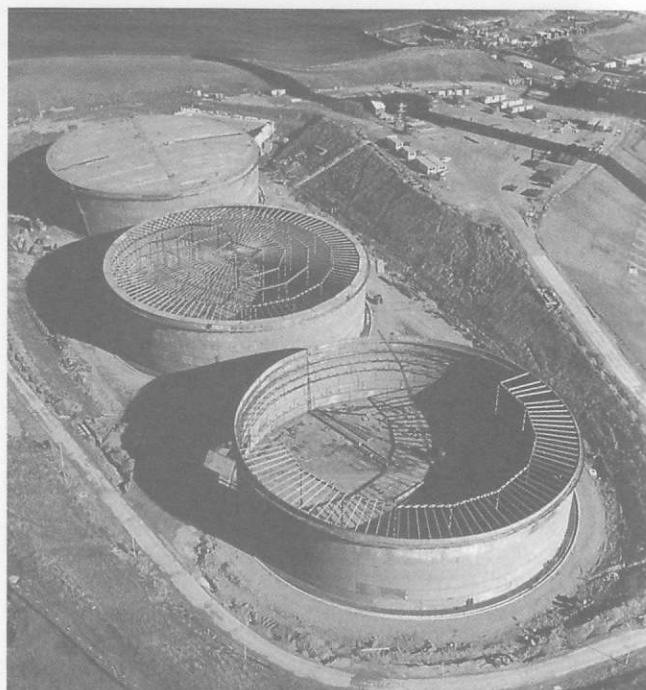
Figure 5.36 Column-supported cone roof tanks under construction Courtesy of Whessoe
