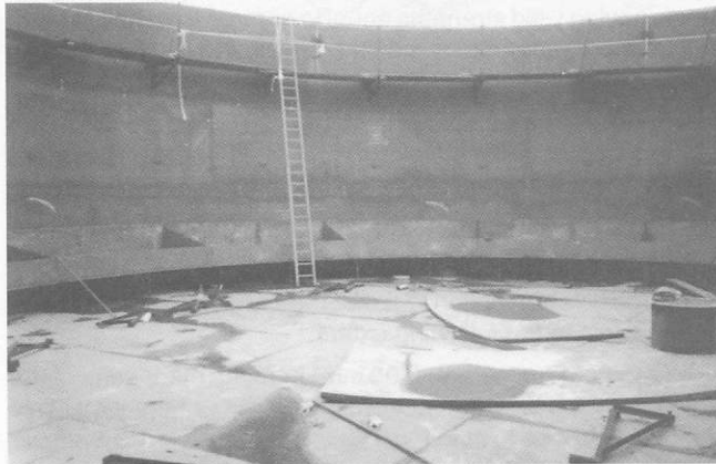
Figure 12.29 20 m diameter single deck roof pontoons being erected on "pins" Courtesy of McTay
