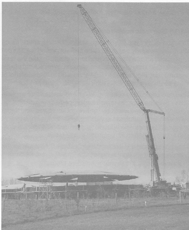
Figure 5.33 A 33 m diameter aluminium geodesic dome roof being lifted into position on a tank Courtesy of McTay
