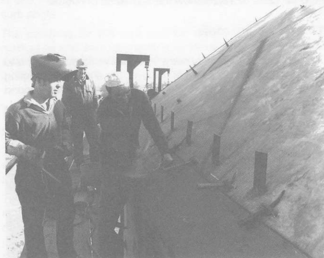
Figure 12.25 The dome roof being secured prior to final welding
