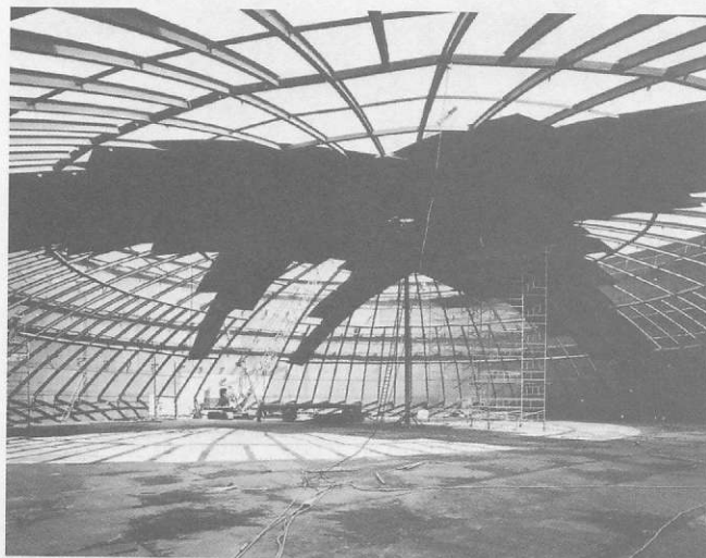
Figure 12.22 31 m diameter dome roof under construction
