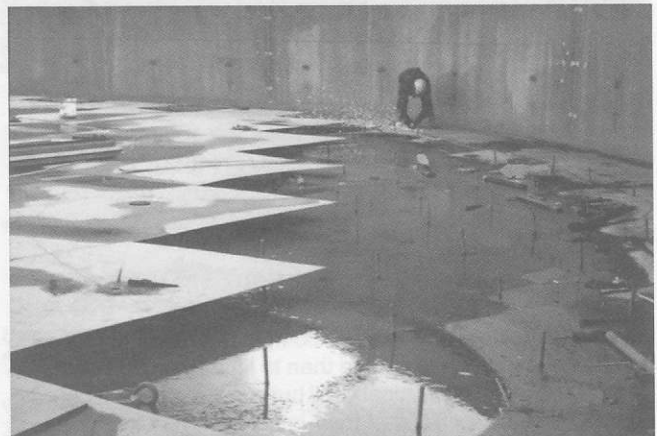
Figure 12.26 Laying the bottom deck of a 36 m diameter double deck floating roof Courtesy of McTay
