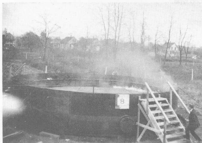
Figure 6.1 CB & I Floating Roof fire test in 1923 Courtesy of
