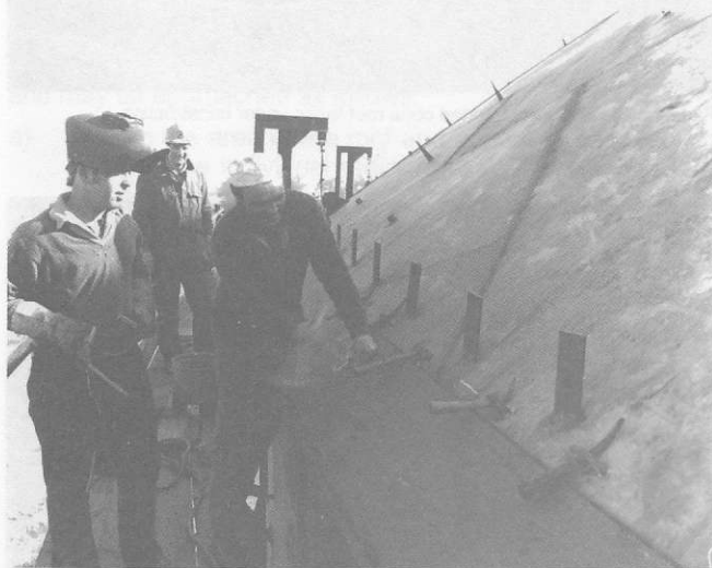
Figure 5.30 A 90 m diameter roof being secured into place
