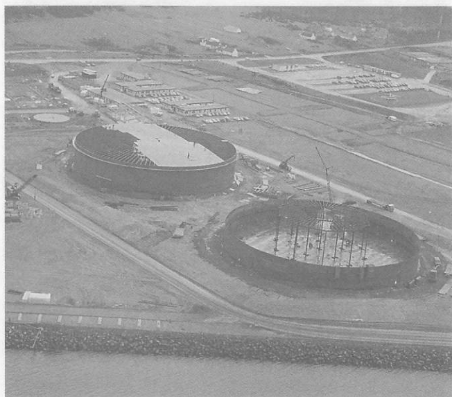
Figure 5.35 Column-supported roof tanks under construction
