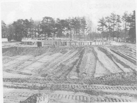
Figure 3.79 The tank roof is clad in reinforced concrete Courtesy of Whessoe
