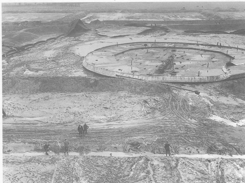
Figure 10.1 The floating roof failure at Fawley in 1952
