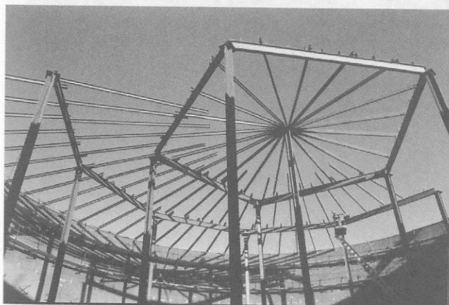
Figure 12.20 A partially erected column-supported roof
