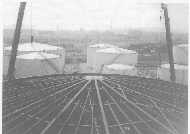
Figure 12.15 Four cranes lifting a 33 m diameter roof structure Courtesy of McTay
