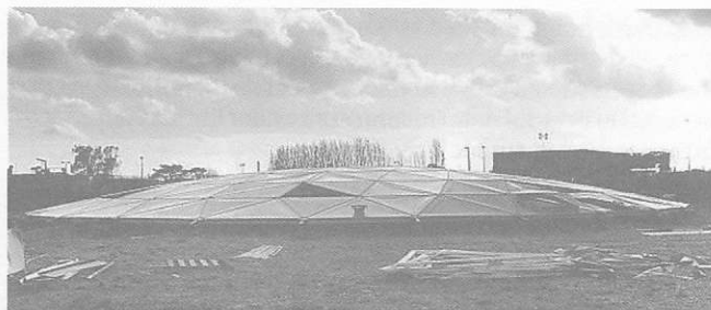
Figure 5.32 33 m diameter geodesic dome roof being built alongside a tank Courtesy of McTay
