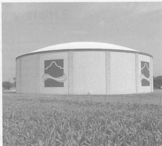
Figure 2.2 Wire-wound concrete water tank Courtesy of Preload Inc
