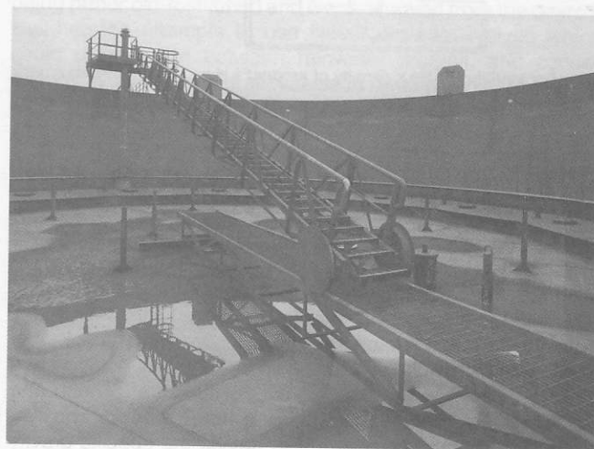
Figure 6.29 Typical rolling ladder with self-levelling treads Courtesy of McTay Engineering
