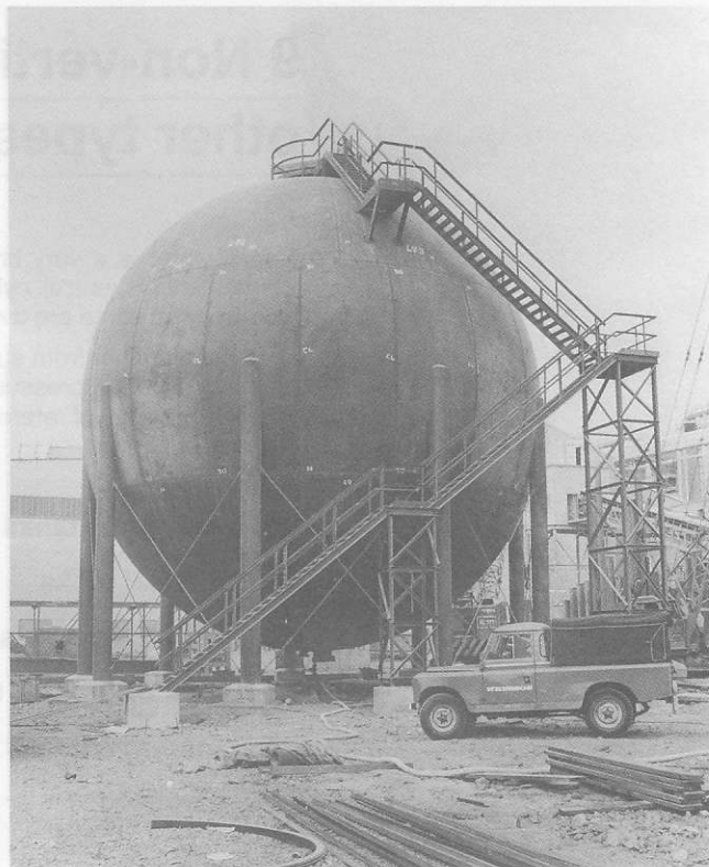
Figure 9.1 A typical spherical tank under construction Courtesy of Whessoe
