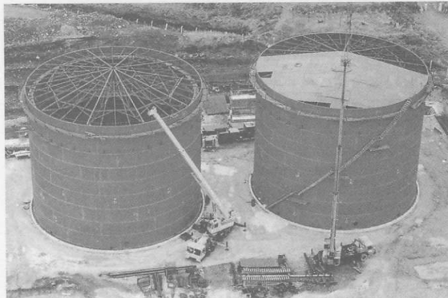
Figure 12.16 Two 25 m tanks nearing completion Courtesy of McTay
