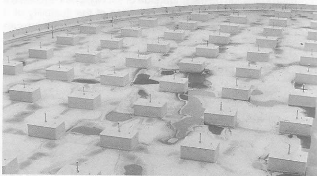
Figure 6.8 A typical buoy roof
