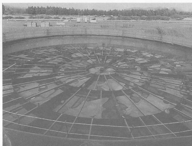
Figure 6.6 A double-deck floating roof under construction Courtesy of McTay
