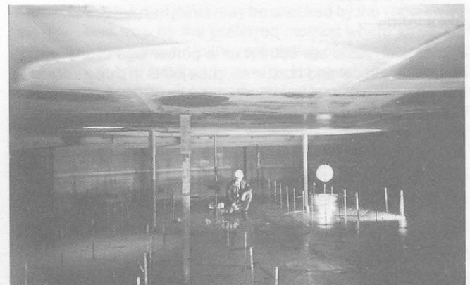
Figure 12.32 20 m diameter single deck floating roof, at its correct elevation (the original support pins can now be removed) Courtesy of McTay
