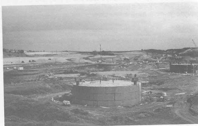
Figure 3.74 Semi-buried tanks under construction Courtesy of McTay
