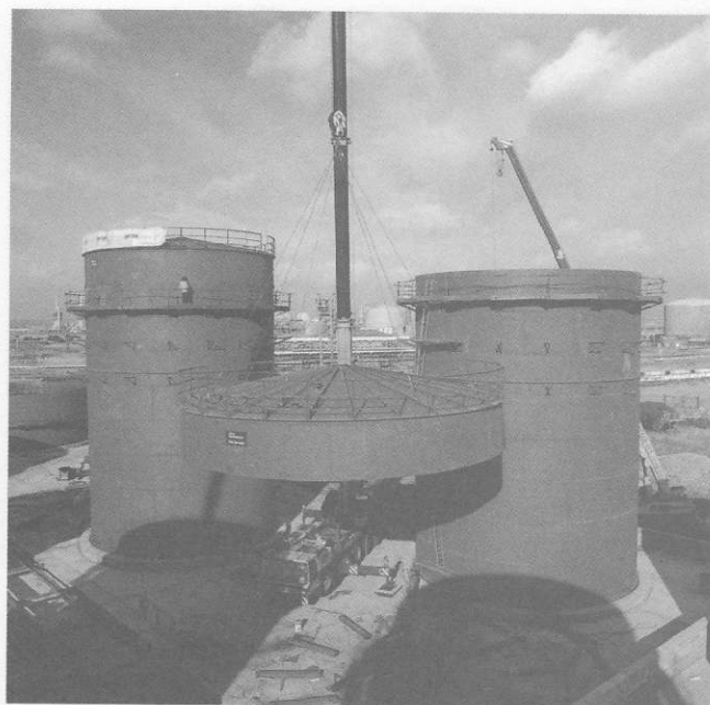
Figure 12.21 A pre-fabricated top section being lifted into place Courtesy of McTay
