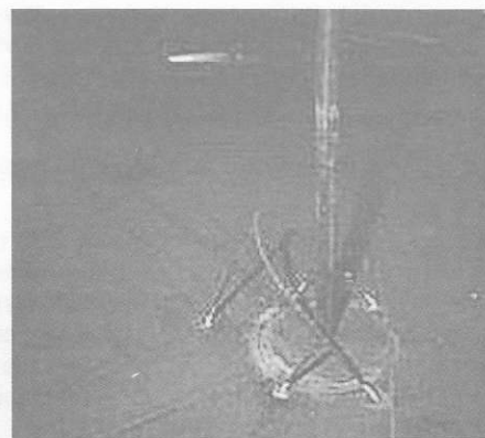
Figure 6.24 A tubular frame welded to the tank floor Courtesy of McTay
