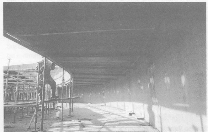
Figure 12.33 A 45 m diameter single deck roof supported off scaffolding Courtesy of McTay
