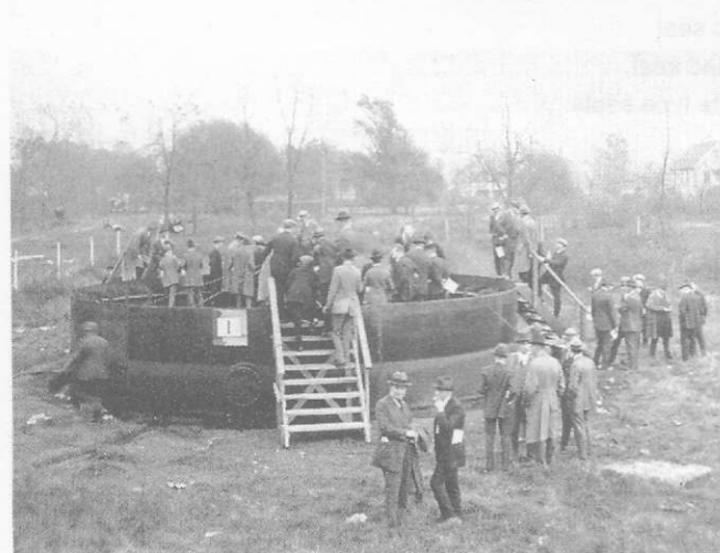
Figure 6.2 CB & I Floating Roof fire test for invited audience of petroleum industry leaders — hats compulsory! Courtesy of
