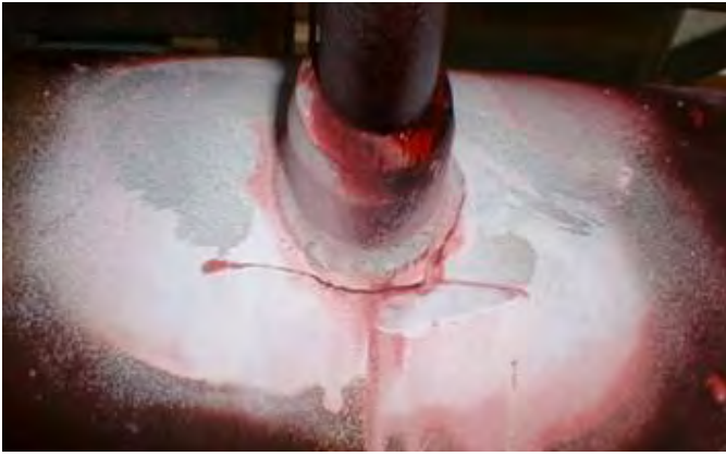
Figure 2-7 An example of a fatigue crack, shown by dye penetrant testing
