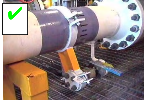
Good SBC bracing to parent pipe
