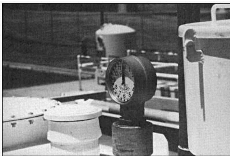
Figure 18 This tank is equipped with a direct-action emergency vent. The vent is immediately left of the clock liquid-level gauge.
