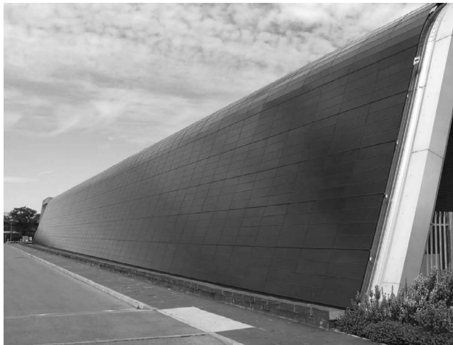
FIGURE 1.2 The 85 kWp Technium OptIC building in St Asaph, Wales, which is covered with the of CIGS modules manufactured by Shell Solar.
