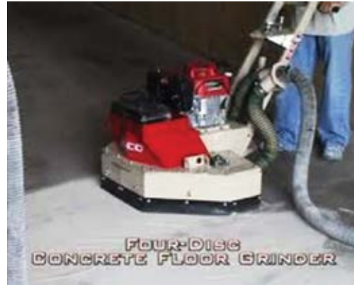
Fig. 8.5.c: Floor grinding with vacuum
