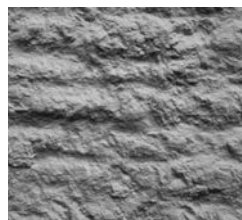
Fig. 6.9: CSP 9 (heavy scarification— rotomilled)
