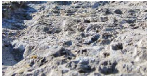
Fig. 8.3.d: Chipped surface using handheld concrete breaker before additional surface preparation
