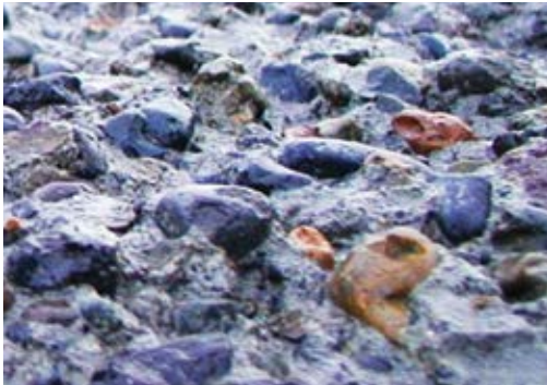
Fig. 6.12: CSP 10—Surface prepared using high-pressure water jetting
