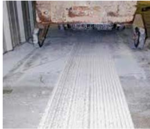
Fig. 8.11.c: Scarified surface showing teeth marks
