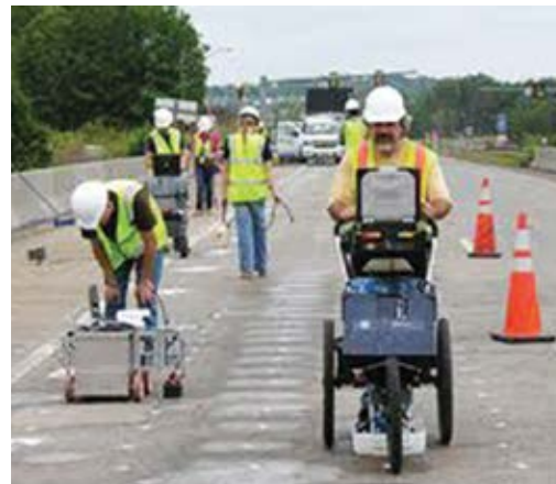
Fig. B.10.a: Electromechanical sounding device
