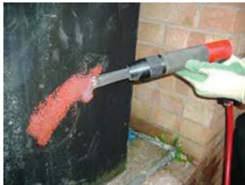
Fig. 8.9.d: Metal surface preparation
