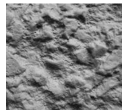
Fig. 6.10: CSP 10 (handheld concrete breaker followed by abrasive blasting)
