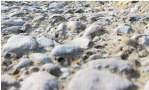
Fig. 6.11: CSP 10—Surface prepared using handheld concrete breaker followed by abrasive blasting
