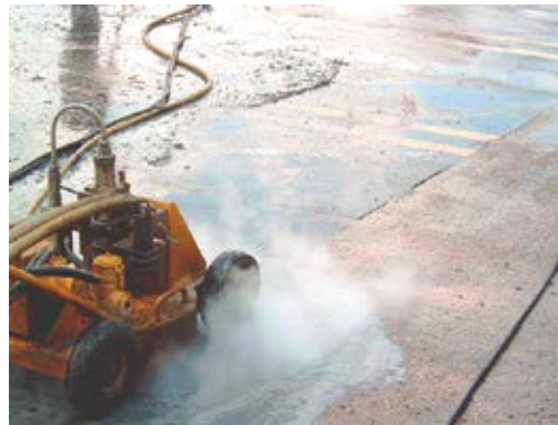
Fig. 8.6.d: Membrane removal—mower
