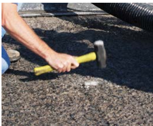
Fig. B.10.c: Sounding using a hammer
