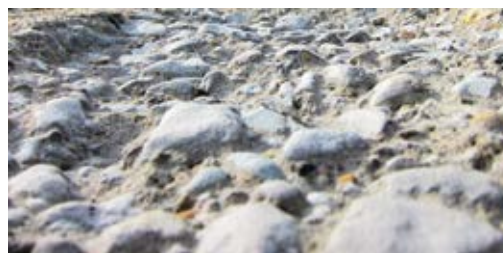
Fig. 8.3.e: Chipped surface followed by abrasive blasting to remove fractured substrate
