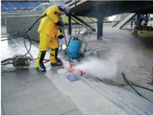
Fig. 8.6.a: Surface preparation—handheld lance
