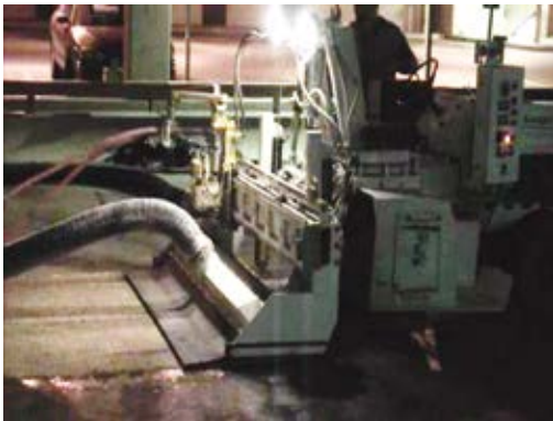
Fig. 8.6.b: Coating removal—robotic equipment
