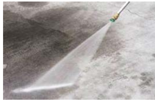
Fig. 8.2.d: Rinsing to remove acid
