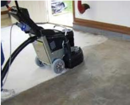
Fig. 8.5.a: Floor grinding
