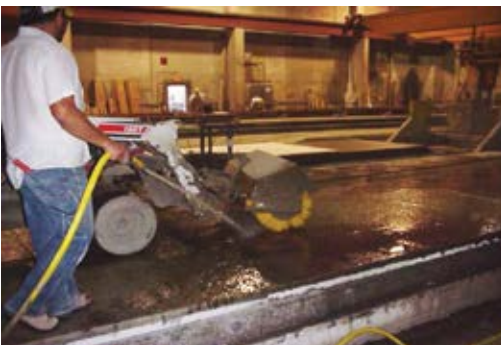
Fig. 8.13.b: Removal of retarder using broom and rinse water
