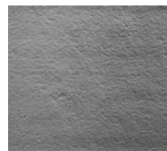
Fig. 6.3: CSP 3 (light shotblast)
