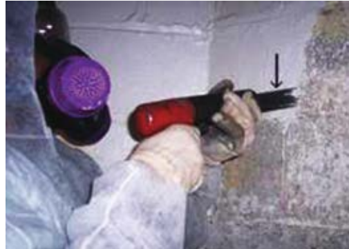
Fig. 8.9.c: Masonry surface preparation
