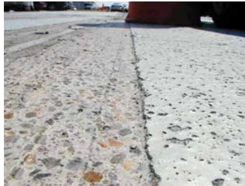
Fig. 8.8.d: Rotomilling used to remove membrane
