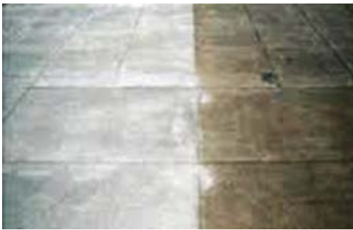
Fig. 8.2.b: Acid applied to concrete
