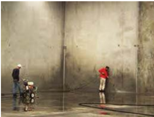
Fig. 8.7.a: Wall and floor cleaning
