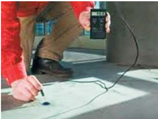
Fig. B.12.d: Installing a moisture probe
