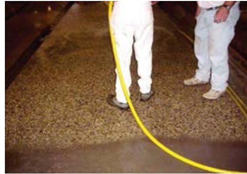
Fig. 8.13.c: Rinsing of exposed surface
