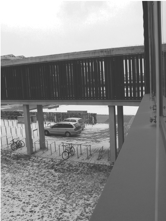
Figure 4.46 Outdoor connection hallway between buildings, south side. A similar hallway leads to shading of the north window.
