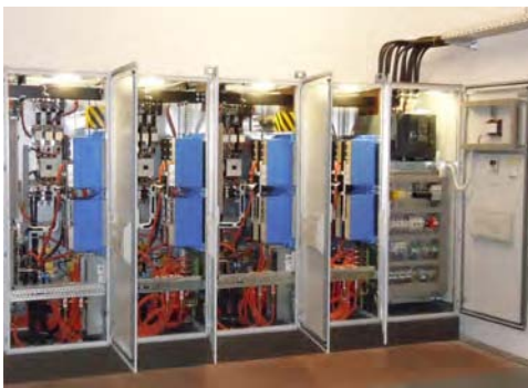
Figure 2.52: ITN-3 converter with 4 outputs (Source: IAS GmbH)
