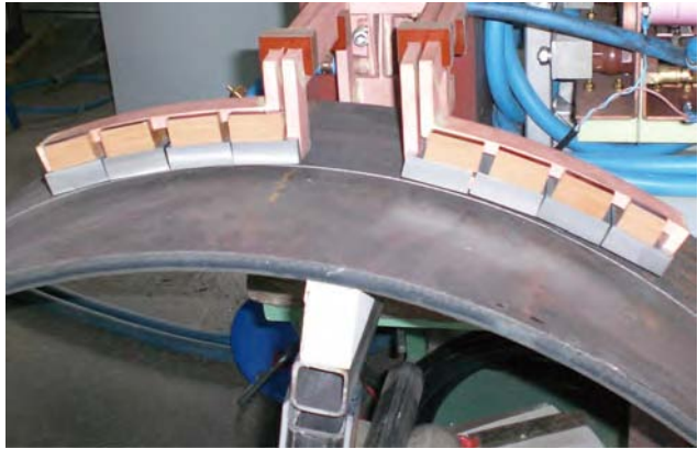
Figure 4.29: Induction assisted orbital welding of tubes
