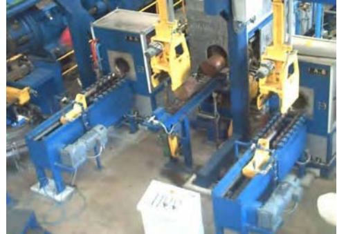
Figure 2.45: Example of a copper billet heating plant with gas pre-heating and two downstream single-billet induction furnaces (Source: IAS GmbH)
