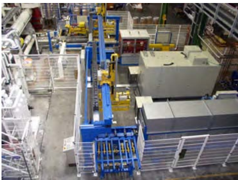
Figure 2.41: Example of a 45 MN press line with upstream gas furnace and billet manipulator (the separate billet delivery system can be seen in the foreground) (Source: IAS GmbH)
