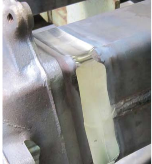
Figure 4.51: IPS outer weld seam
