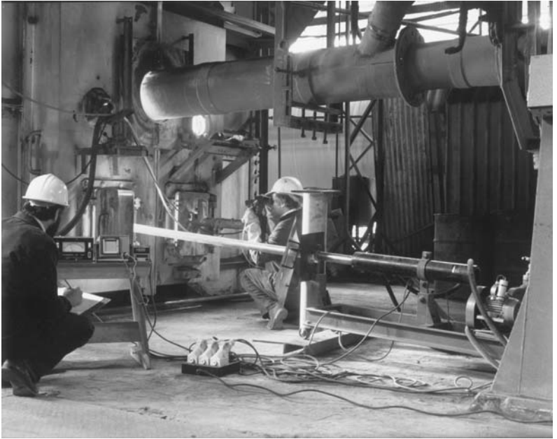
Figure 9.4 Plant trials using a suction pyrometer to measure combustion air temperature and an optical pyrometer to measure product discharge temperature
