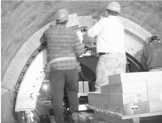
Figure 11.6 Tapered brick being installed in a rotary kiln; note the purpose built support frame to facilitate quick and accurate installation (photo courtesy of Brokk Bricking Solutions Inc.)
