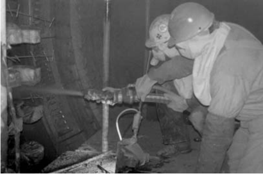
Figure 11.9 Gunning refractory into place in a rotary kiln (photo courtesy of REED Gunite Equipment)
