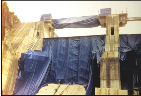
Containment on Dam Gate
