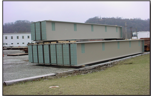
Masked areas at bolted connection points
