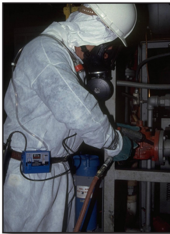
Worker properly protected
