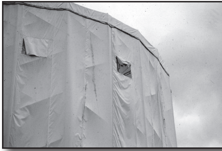
Containment under negative pressure
