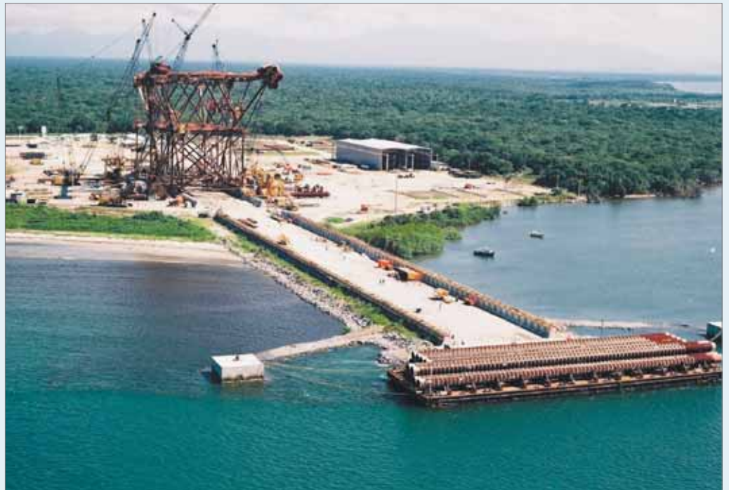
Figure 1. Overview of the Techint construction site in Pontal do Paraná/Parana at the time of the construction of the PRA-1 jacket.
