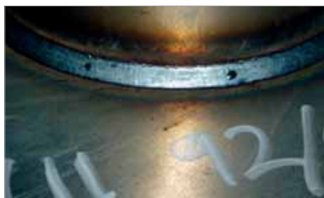
OK Tubrod 14.11-1.2mm in 92%Ar/% CO 2 –Torch angle 20° pushing. Pipe to plate connection.
