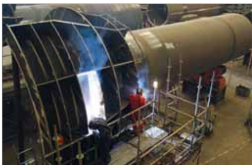
Figure 4. FCAW of the sleeves – the part that catches the foundation pile.
