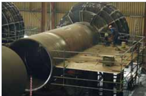
Figure 5. Submerged arc welding of a sheer plate onto a pile sleeve.
