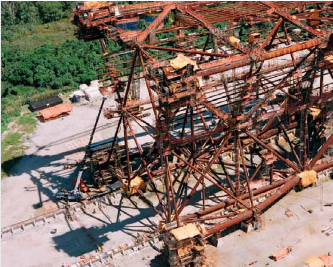
Figure 2. Overview of the jacket in its final assembly phase.
