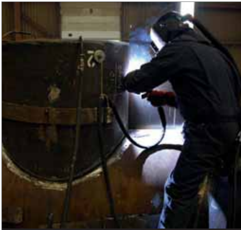
Figure 8. FCAW of a lifting trunnion.
