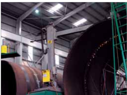
Figure 4. Filling and capping the remaining V-joint from the outside. Preheating by means of oxyfuel burners.
