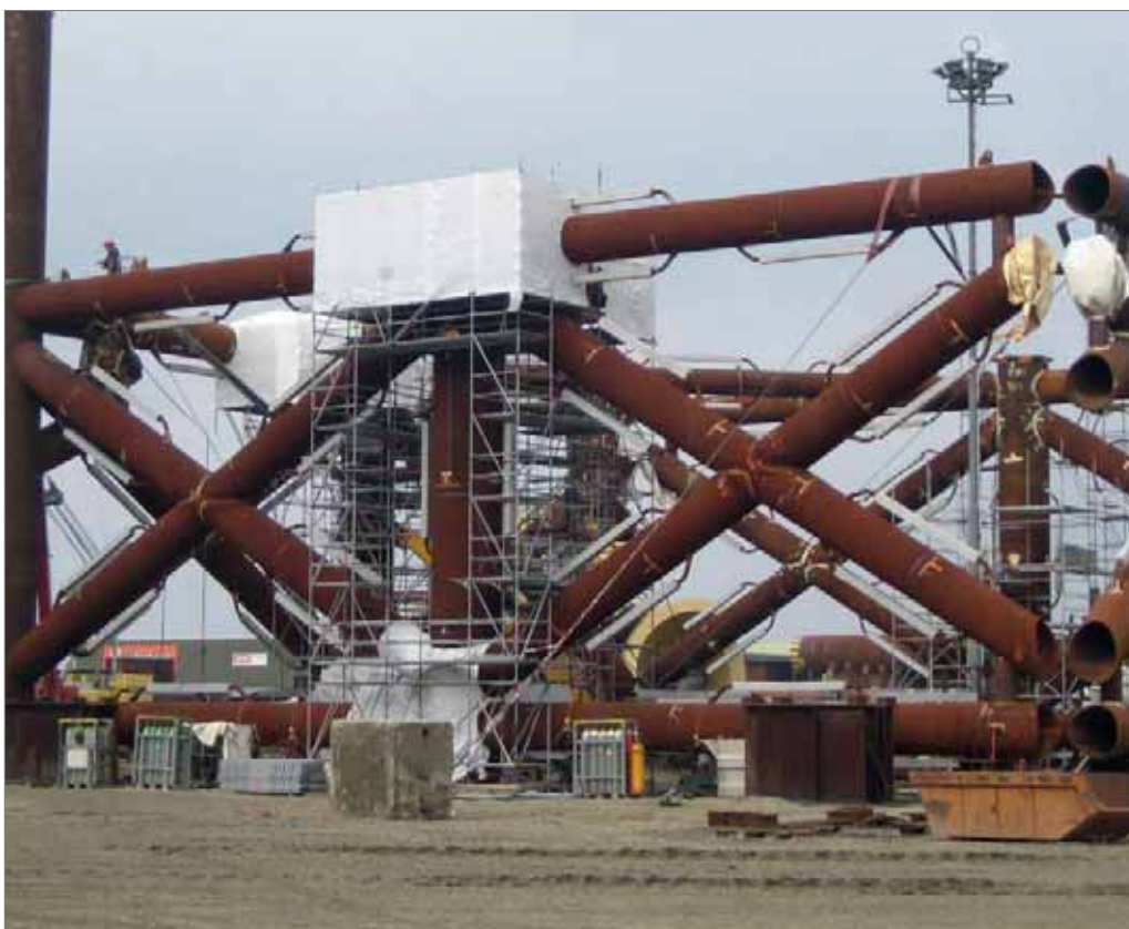
Figure 7. Erection of the template. All rows are first carefully positioned within the tolerances – with the help of temporary columns (left) – before they are attached to the docking pins in the pile sleeve cluster (cluster visible in the background).
