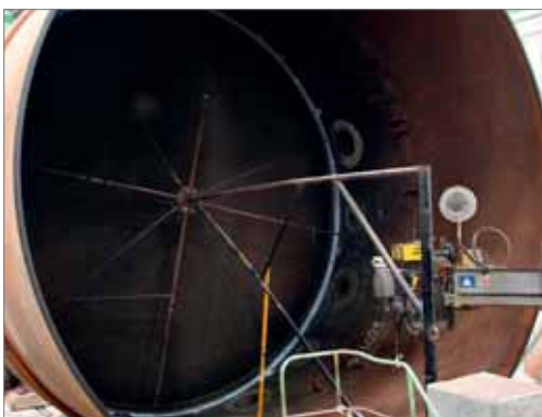
Figure 3. Single wire narrow gap SAW from the inside of the reactor.
