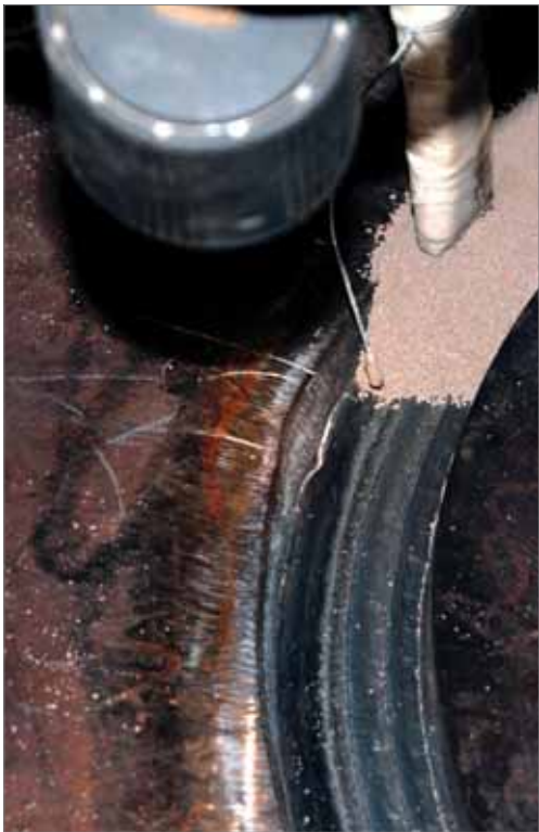
Figure 7. Automatic SAW of a nozzle.
