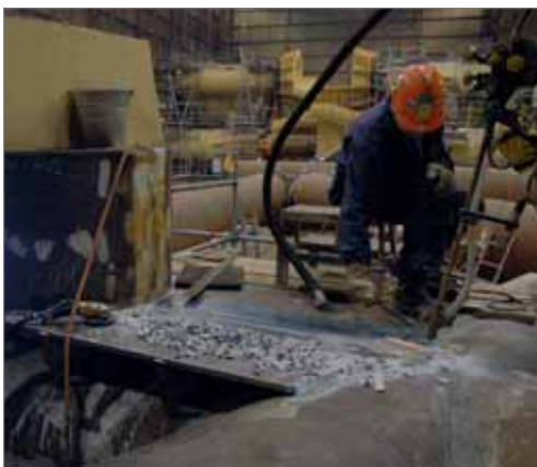
Figure 9. SAW on a lifting trunnion.
