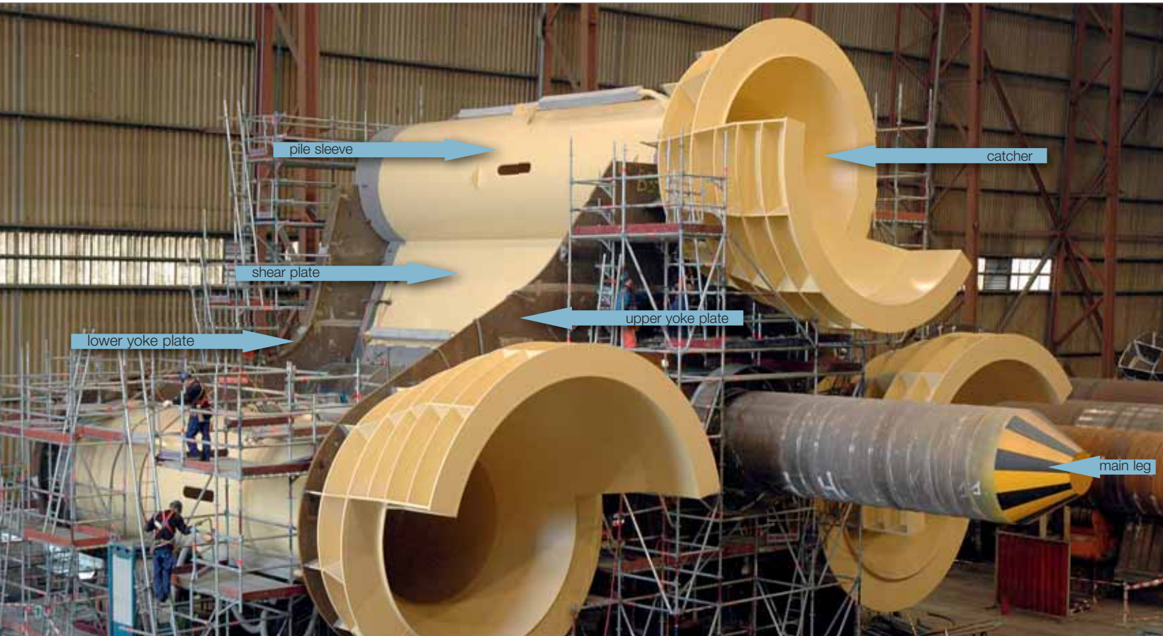
Figure 3. Fabrication of a pile sleeve cluster.
