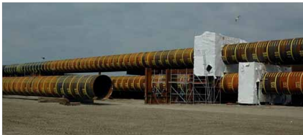
Figure 10. Welding tents made from shrink foil protect the weld area from wind and rain.
