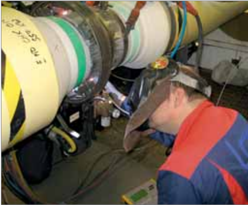
Figure 2. Vertical-down welding of a flowline in super-martensitic stainless steel, using orbital TIG welding equipment. The operator can control the welding parameters without lifting his helmet.
