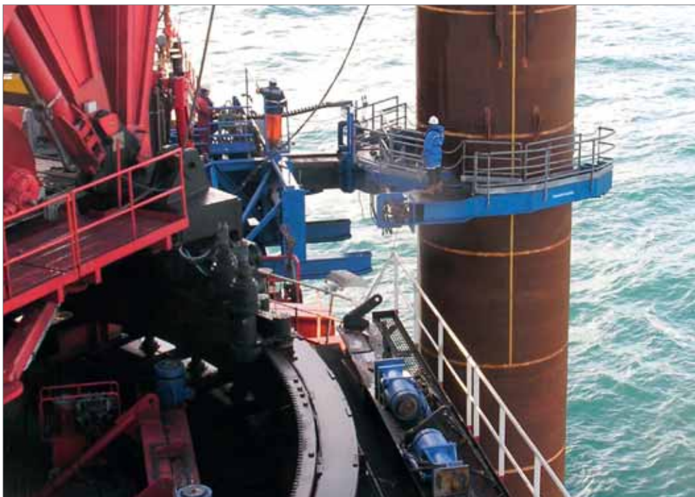
Figure 1. One of the monopiles being driven into the sea bed. The piles are 50 or 54 m in length and the water depth is 19-24 m. Source: Offshore Windpark Q7.
