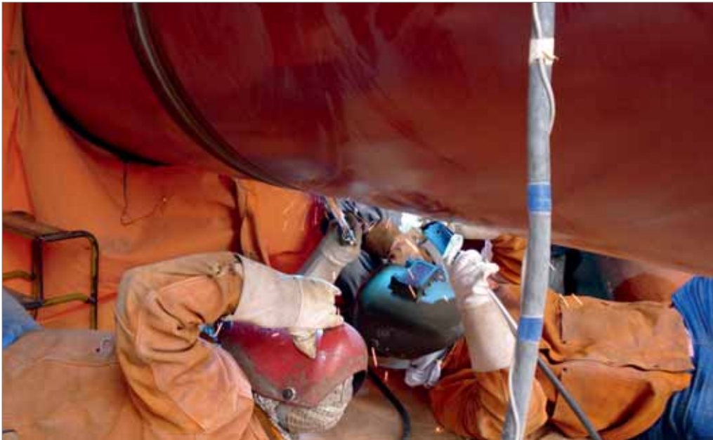
Figure 2. STT root pass welding
