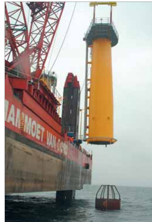
Figure 2. Positioning of a transition piece onto a monopile. The transition piece reaches 15 m above sea level.
