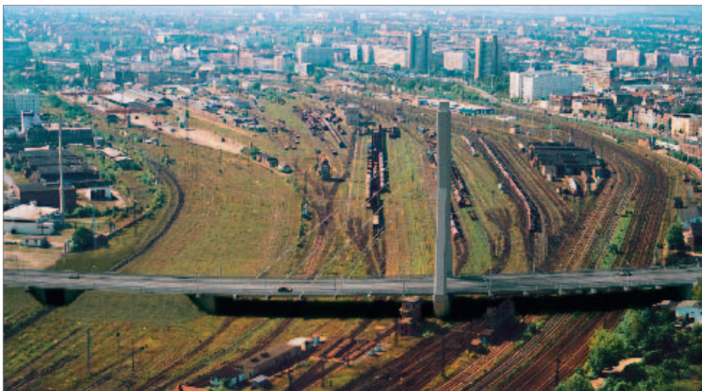
The new Berliner Bridge
