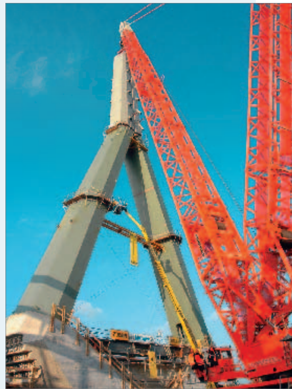
Figure1. Erection of the 73 metre tall, all steel pylon.
