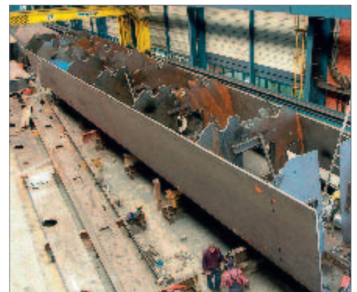
Figure 6. Assembly of the pylon's outer plates.
