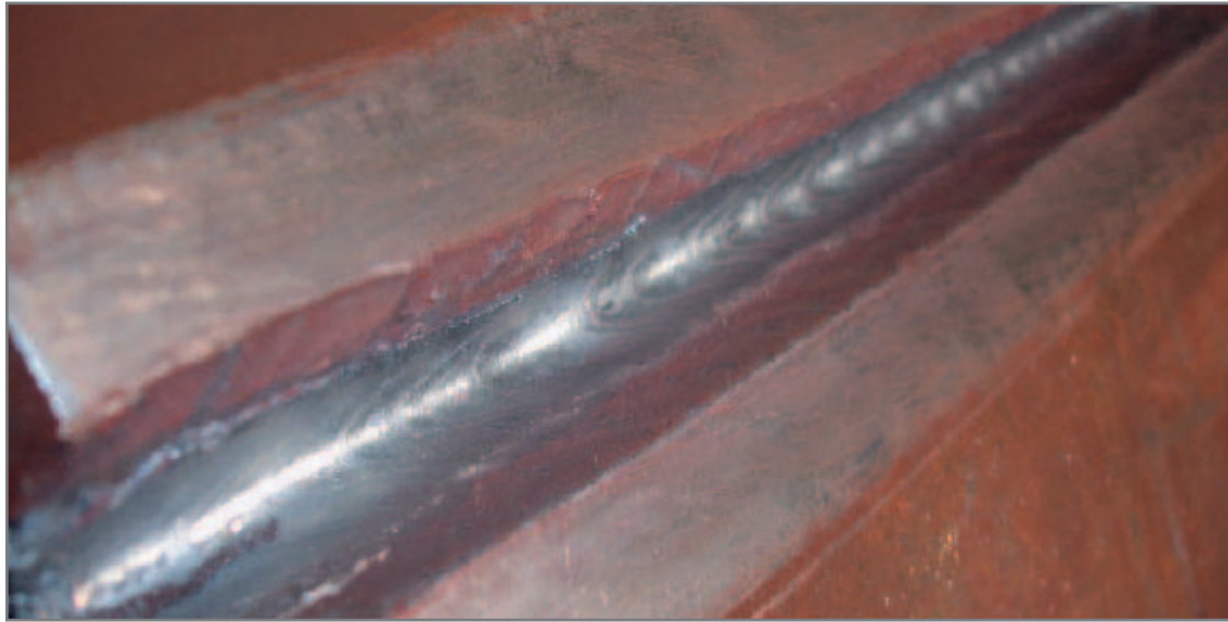
ESP-150 plasma gouging used for the removal of weld defects in the manufacturing of large tubes.
