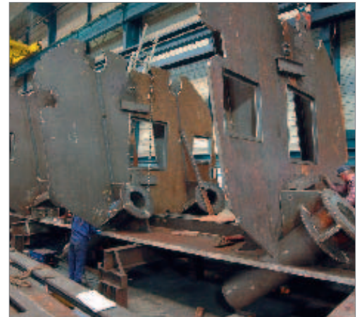
Figure 5. Assembly of the bulkheads and anchoring tubes.
