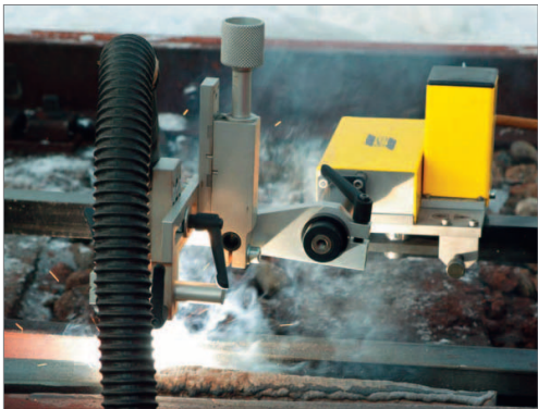
Figure 2. ESAB Railtrac BW1000 equipment used for hardfacing the rail heads of a crossing with OK Tubrodur 15.43. It is lightweight equipment – programmable with a control unit and operated by remote control. Shown here is the Railtrac BV1000.
