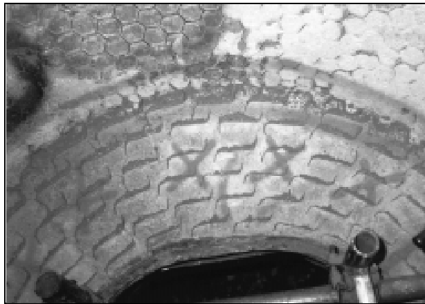
Fig. 2800-4 Unidentified Area Showing Loose Refractory Biscuits—Hexmesh was incorrectly installed and formed narrow gaps which were impossible to pack properly. Replace both hexmesh and refractory.
