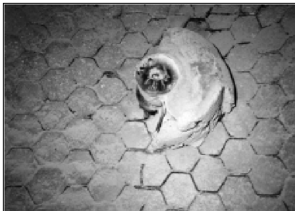
Fig. 2800-5 FCCU Regenerator U-bend—Erosion of Aeration Nozzle—Chop out and replace nozzle refractory. Metal of surrounding hexmesh shows, but this is acceptable. No anchorage repair needed.
