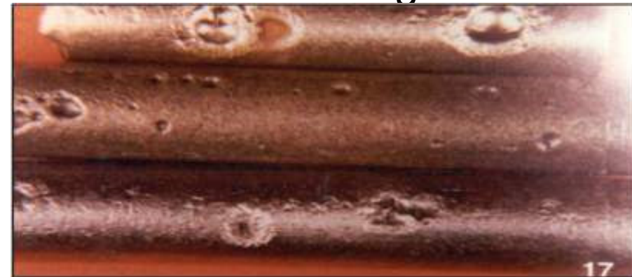
H 2 S Pitting
