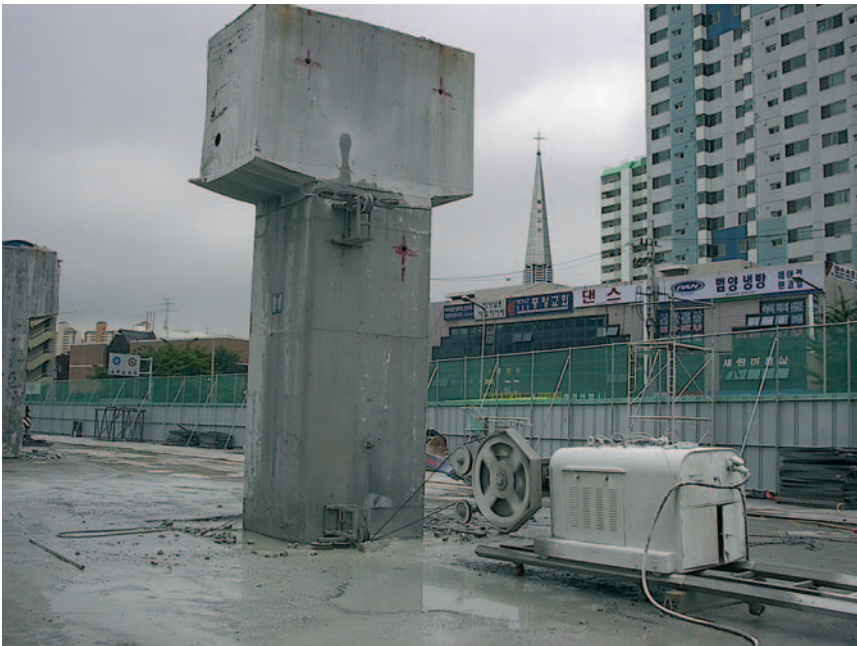
Figure 8.10 Diamond wire saw cutting a reinforced concrete pile into small sections to facilitate its removal. (Courtesy of EHWA Diamond Ind. Co., Ltd.)
