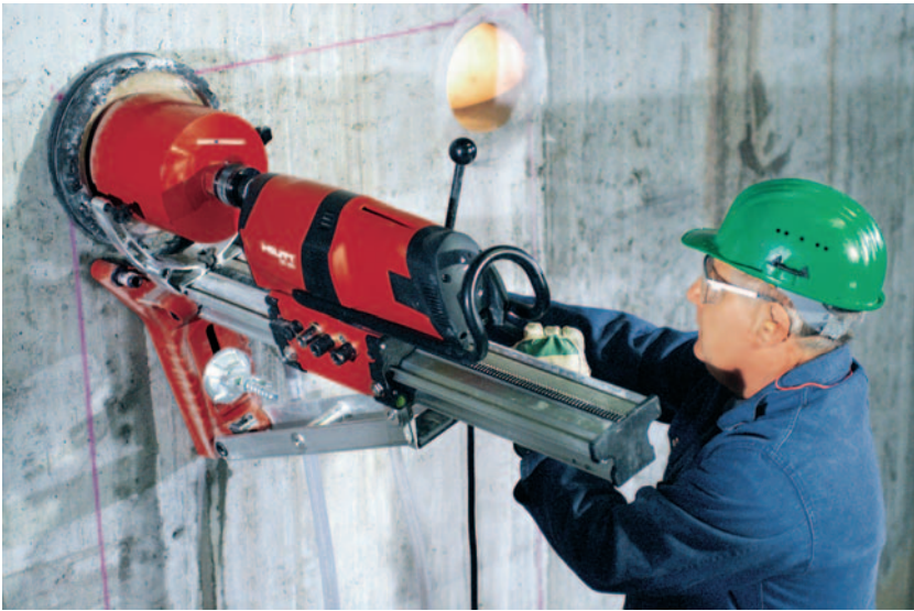
Figure 8.12 Portable drill rig mounted for drilling through a concrete wall. (Courtesy of Hilti Corporation)
