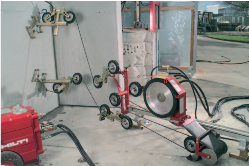
Figure 8.9 Portable wire machine making a vertical cut in a concrete wall. (Courtesy of Hilti Corporation)
