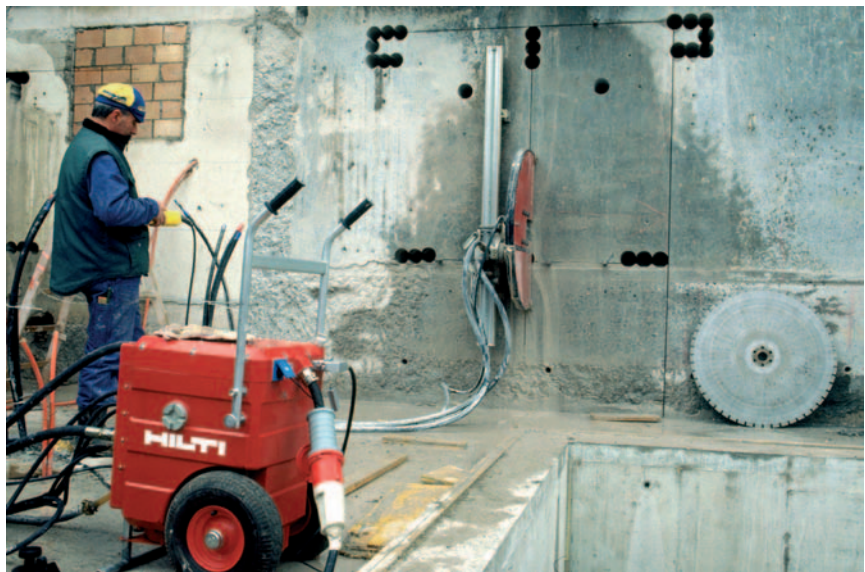
Figure 8.3 Remotely controlled wall saw cutting a doorway in a concrete structure. (Courtesy of Hilti Corporation)
