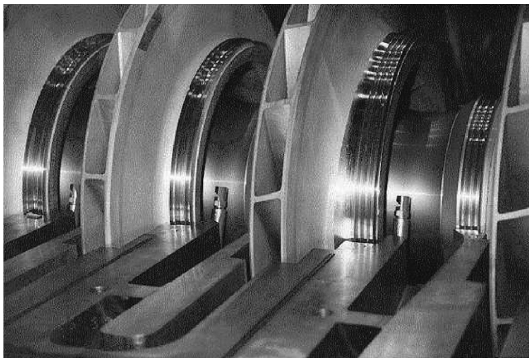
FIGURE 8.4 Nozzles installed for on-line washing of compressor rotor.
