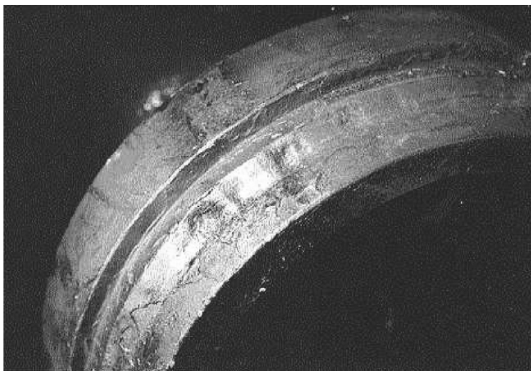
FIGURE 8.1 Coke deposit on the plug of a globe valve.
