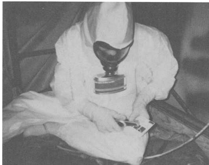
FIG. 2—Calibrating a dry film thickness gauge (courtesy of Stone & Webster Engineering Corp.).
