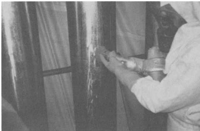
FIG. 27—Vacuum blast operation (courtesy of Stone & Webster Corp.).
