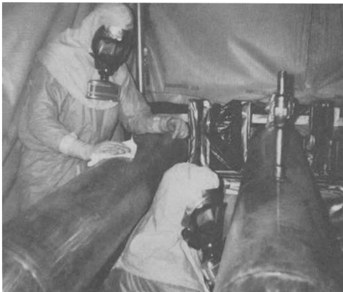
FIG. 19 —Solvent cleaning (courtesy of Stone & Webster Engineering Corp.).
