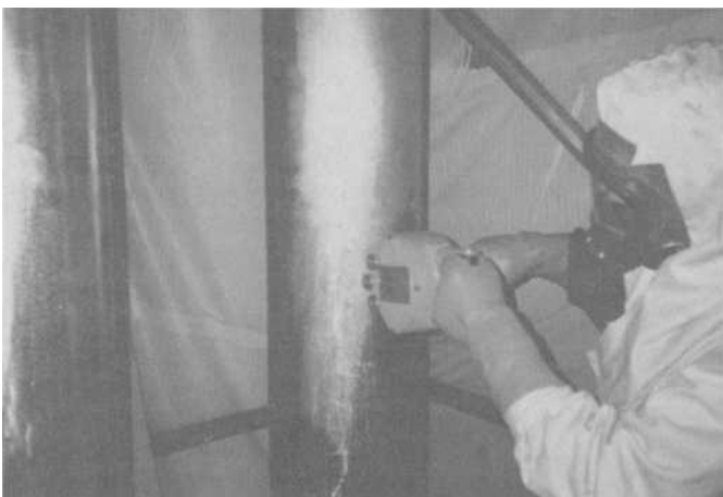
FIG. 25—Rotary impact tool operation (courtesy of Stone & Webster Corp.).
