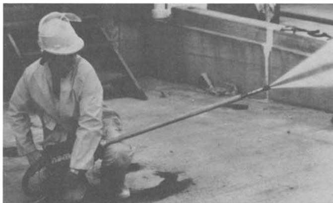
FIG. 28—ADMAC high-pressure water blasting equipment (courtesy of KTA-Tator, Inc.).
