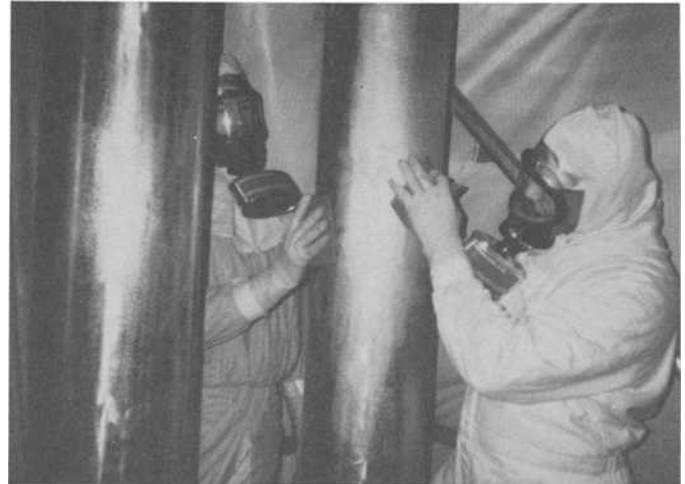
FIG. 20 —Hand tool cleaning (sandpaper) (courtesy of Stone & Webster Corp.).
