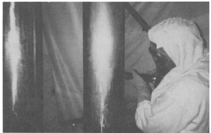
FIG. 22 —Needle gun operation.
