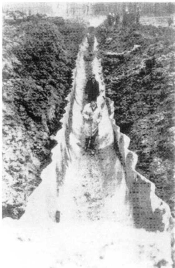
Figure 5.19 - Ductile fracture of large diameter line pipe showing scalloped fracture edges. 2 (Reprinted with permission from Sixth Symposium on Line Pipe Research, October 1979. Research sponsored by the Pipeline Research Committee, American Gas Association, Arlington, VA)
