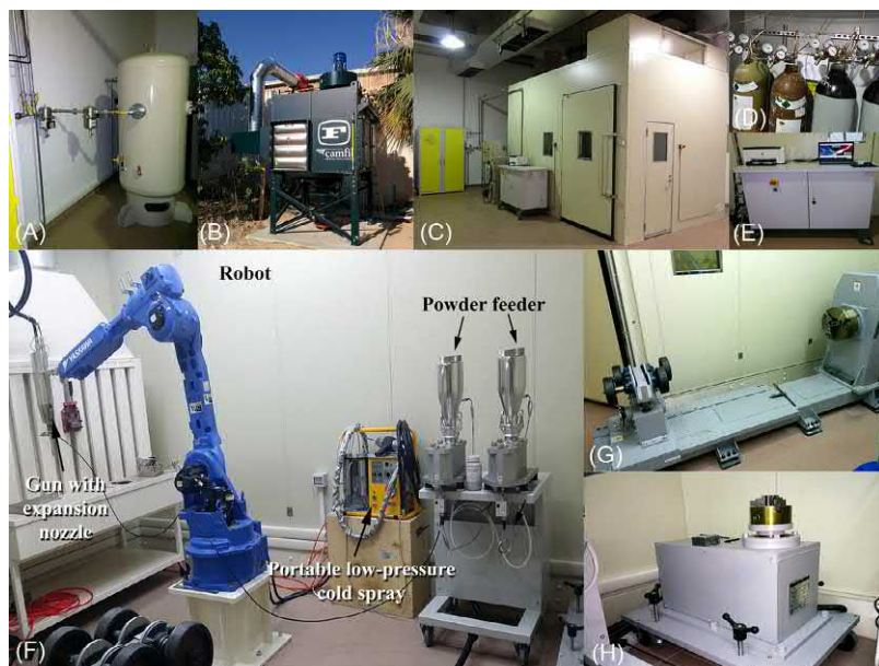
Figure 12.8 Photos taken from the Nanotechnology Laboratory, Energy and Building Research Center (EBRC), Kuwait Institute for Scientific Research (KISR), present the components of a cold spray system (provided by Startack Co. Ltd., Japan). The system consists of high-pressure air compressor to compress the air in a high-pressure tank (A), a dust collector (B), spray room (C), gas control unit with a gas mixer (D), and central process control unit (E). The component of the system installed inside the spray room including the powder feeder, a robot, and low-pressure cold spray system is shown together in Fig. 12.7F, which carries the gun during the coating process. (The gun with the expansion nozzle can be oriented in a horizontal or vertical positions, as shown in Fig. 12.8A and B, respectively, which is used for outdoor coating that can be also installed and manually operated inside the room (Fig. 12.7F). Horizontal and vertical turntables are displayed in Fig. 12.7G and H, respectively.
