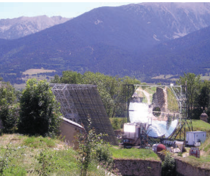
Facilities such as the Mont-Louis Solar Furnace (above) and the Odeillo Solar Furnace (right and on the opening pages) concentrate sunlight to conduct thermochemical experiments.
