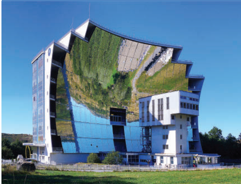
Facilities such as the Mont-Louis Solar Furnace (above) and the Odeillo Solar Furnace (right and on the opening pages) concentrate sunlight to conduct thermochemical experiments.
