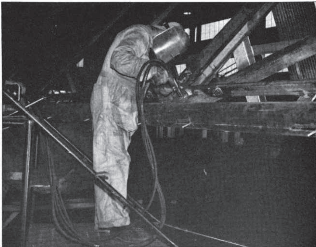
Fig. 6-6. Steel being joined by CO 2 MIG welding. In this process, carbon dioxide gas shields the arc.
