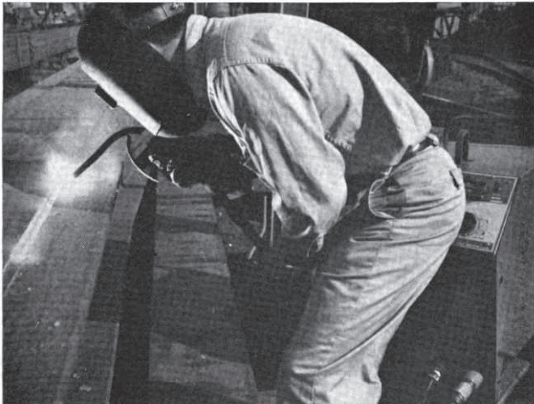
Fig. 6-11. Semi-automatic vapor-shielded welding doubles or triples previous production rates. In outdoor applications, there's no problem with wind blowing shield away from weld. Continuous electrode fed mechanically through the lightweight gun enables welder to follow any joint easily.
