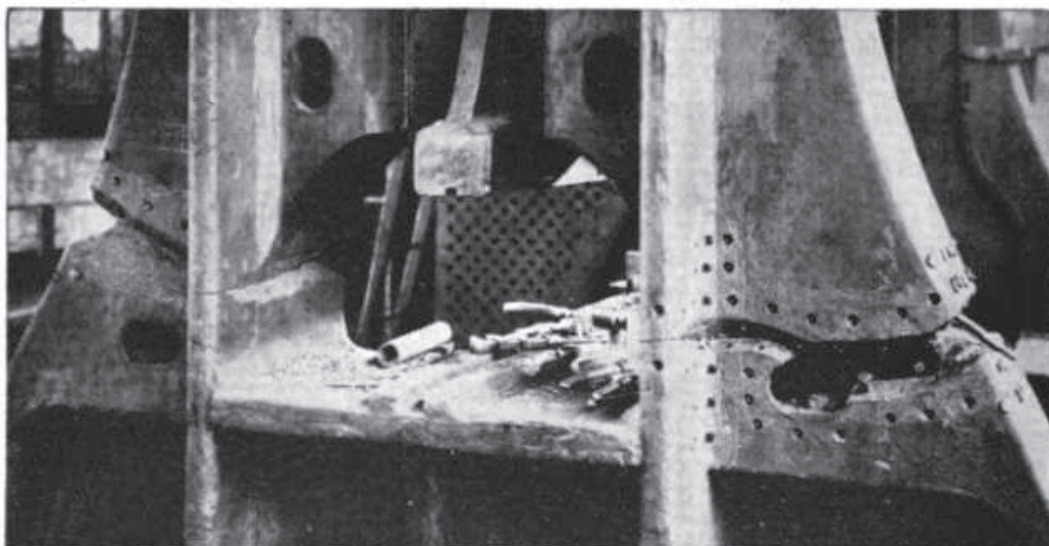
Fig. 14-7. Here the crack has been V'd out, drilled and tapped and some studs are in place.
