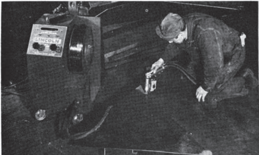
Fig. 6-16. Semi-automatic submerged arc equipment, with which both electrode and granulated flux are fed mechanically, permits greatly speeded production on applications previously requiring manual welding. Here, parts of a power plant flue system are being assembled at double the former welding speeds.
