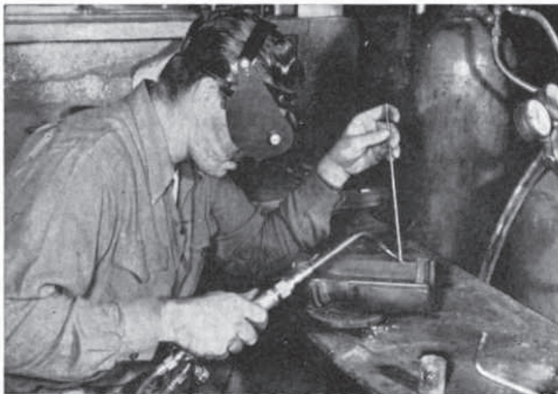
Fig. 6-12. The most common of the gas welding processes is oxyacetylene welding, using a hand-held torch and welding rod.
