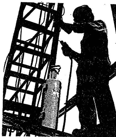
Fig. 8 — Portable Electrode Storage Oven serving on site
