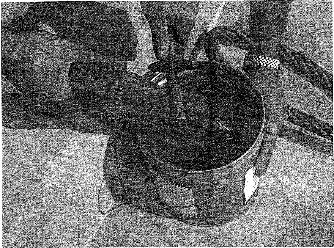
Figure 3-47. Mixing of low viscosity epoxy grout.
