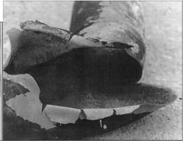
Figure B5c: Failure at Extrados from Downstream Elbow
