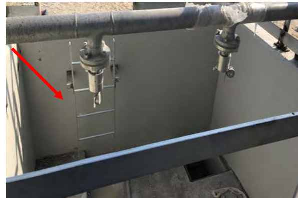
Figure 9B and 9C: Concrete Access Pits (1.8 m to 2 m height)
