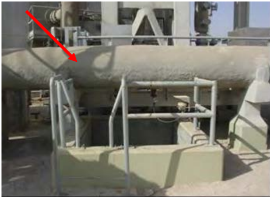
Figure 9B and 9C: Concrete Access Pits (1.8 m to 2 m height)
