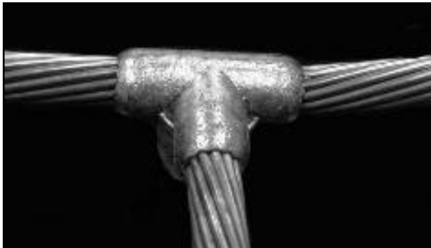
Figure 6. Example of an exothermic weld
