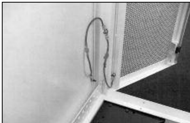
Figure 28. Illustration of a bond connection from a cabinet to the cabinet door
