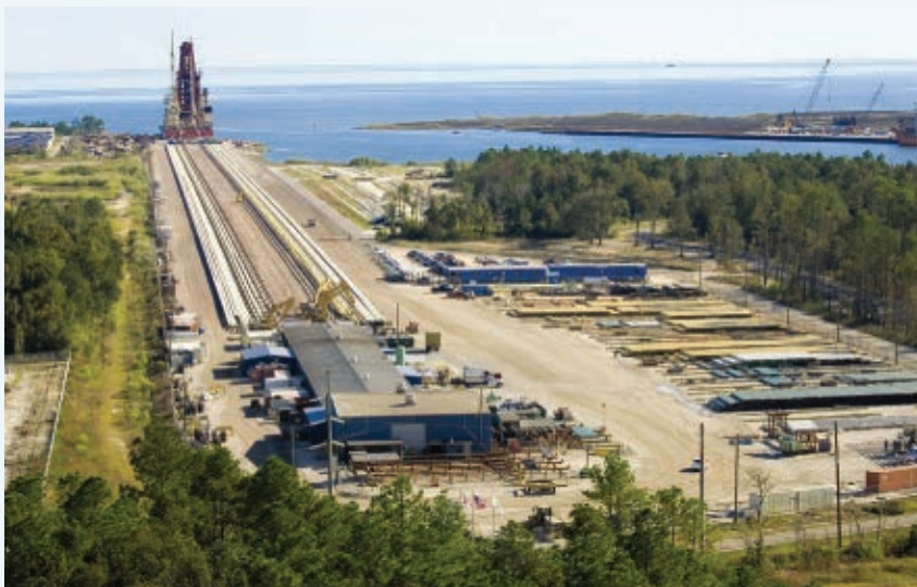
▲ Technip's spoolbase, Mobile, Alabama.
