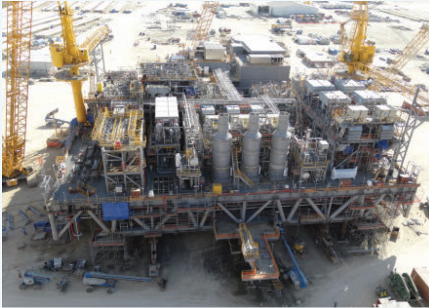
▲ Delta House Topsides Fabrication / Integration being completed at Kiewit Offshore Services.
