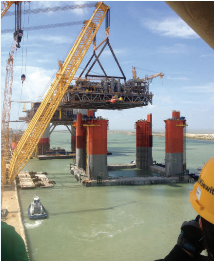
▲ The Delta House topsides are set on to the hull using Kiewit's Heavy Lifting Device (HLD), which has a capacity of 13,000 short tons.
