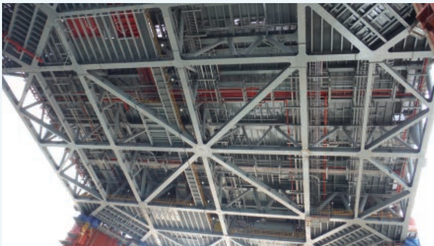
▲ Exmar's single-lift truss deck remains dry in a 1,000 year Gulf of Mexico hurricane.
