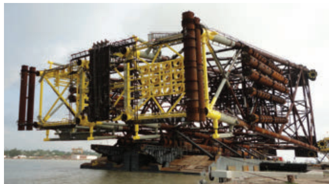
The Ayatsil-A jacket on board the Intermac 600 transportation and launch barge. (Photo courtesy Business Wire)
