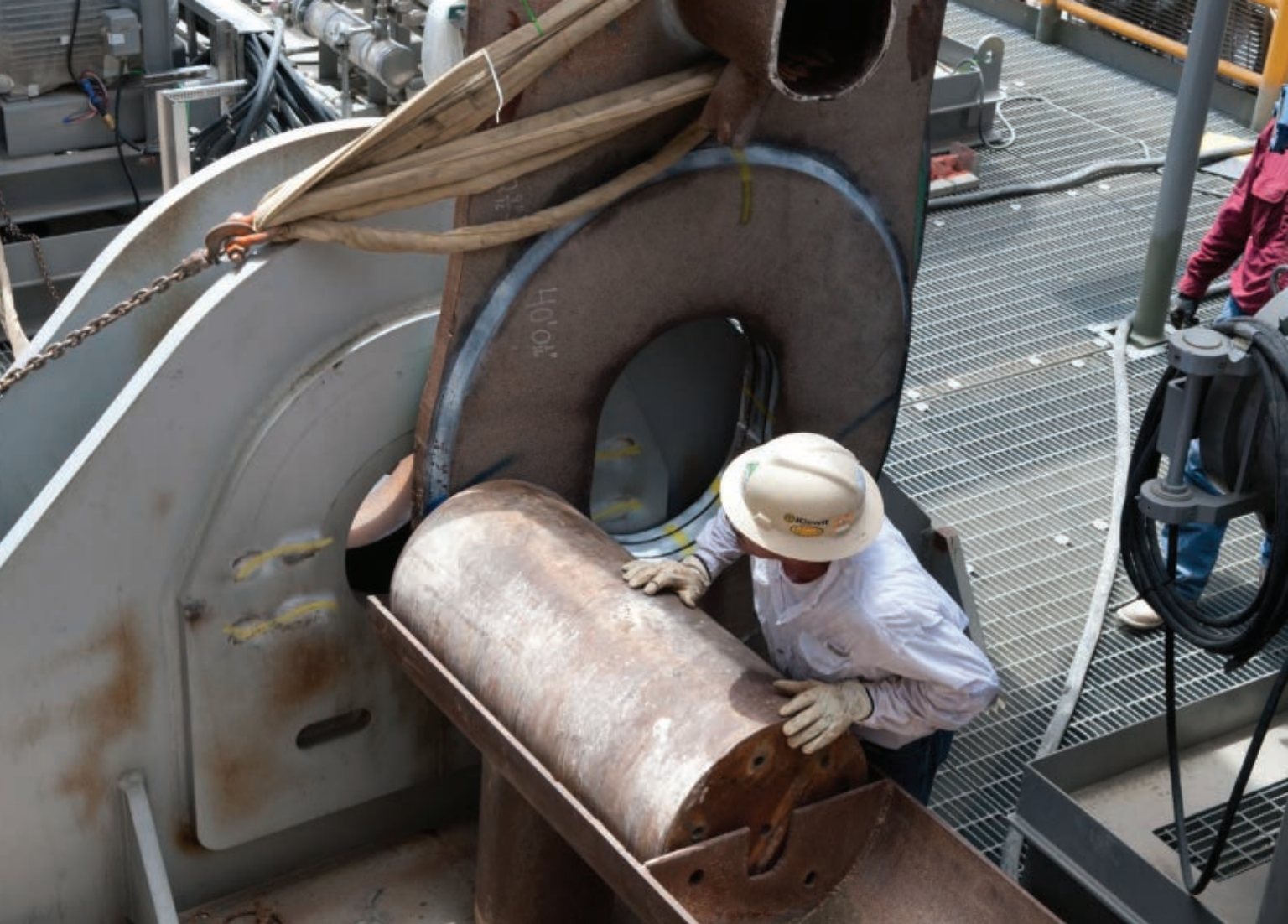
● Massive slings were attached to lift the 9,580 metric-ton Delta House topsides onto the hull.
