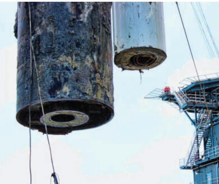
The cutting wire sawed through the mud and cleanly severed the 60-in. caisson along with both internal and external conductors.
