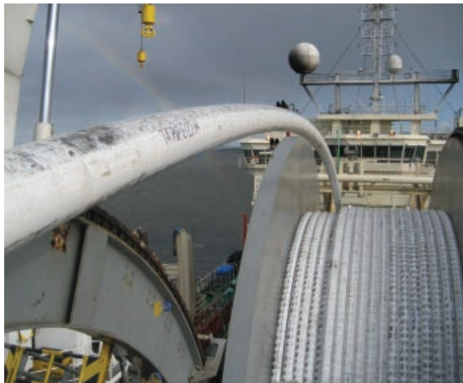
Spooling pipe-in-pipe onboard reel-lay vessel.
