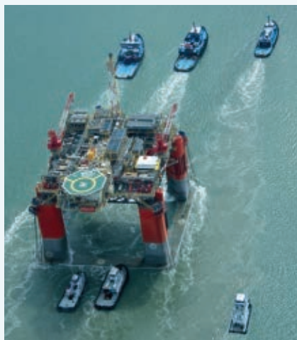
▲ The OPTI® semisubmersible hull is scalable to meet operator needs and is water depth independent. OPTI-EX® installed July 2011 (shown left), and Delta House installed September 2014 (shown right).
