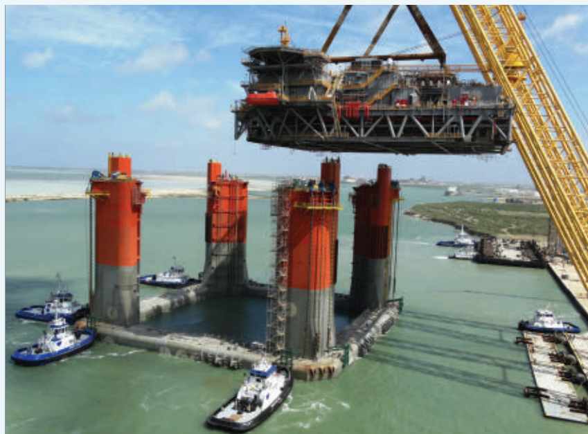
▲ Delta House deck set safely on the hull.
