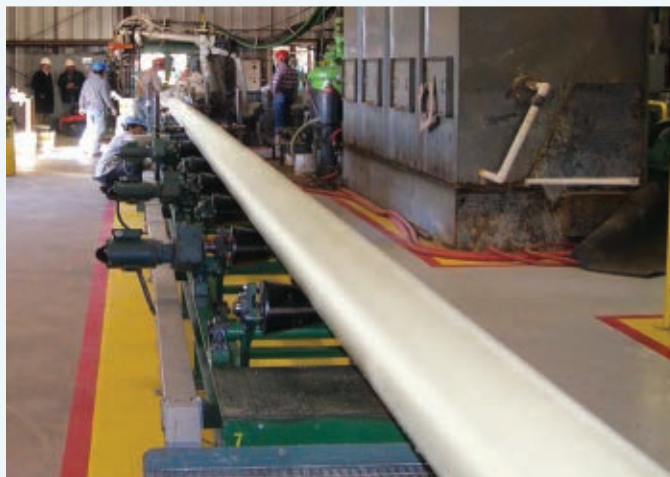
◀ GSPU insulating 80 foot (24m) double joined pipe.
