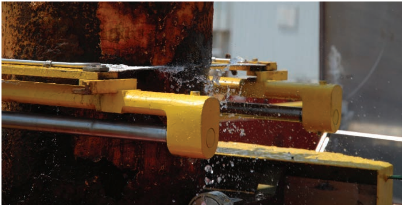
The conductor removal technology has enhanced safety by eliminating manual handling and hot work issues.
