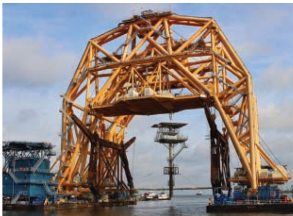
The VB 10,000 lifted the structure and carried it back to port.
