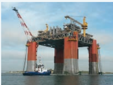
▲ GATE lead pre-commissioning activities of topsides prior to integration with the hull.
