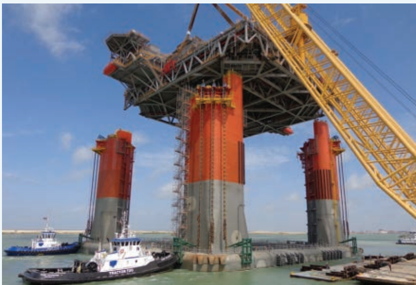
▲ The Exmar OPTI-11,000® single-deck lift set a record of 9,580 tons at Kiewit Offshore Services.
