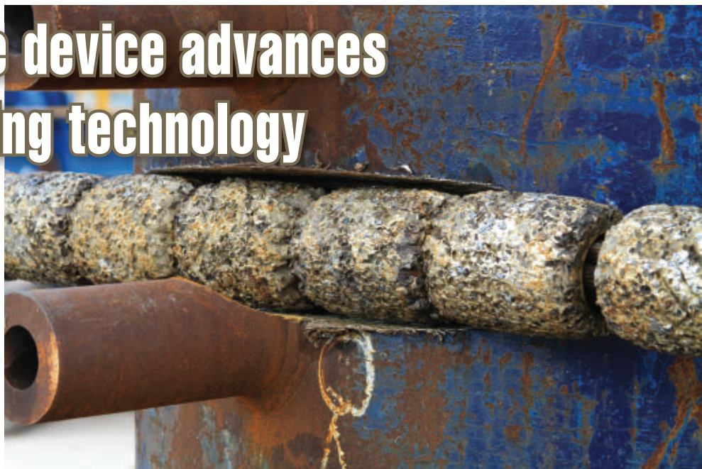
Operated by hydraulic winches, the wire sawed through a pipe 24 in. in diameter with a 2-in. steel wall in less than one hour. (All photos courtesy Versabar)
