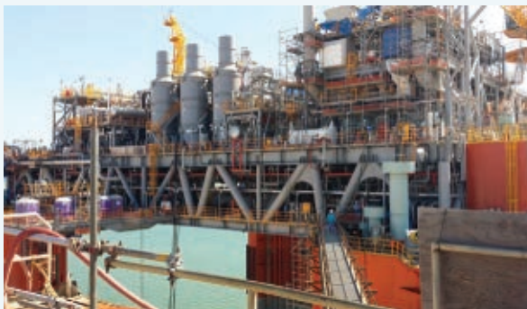
▲ GATE's Systems Approach helped to streamline the Systems Completions Process.
