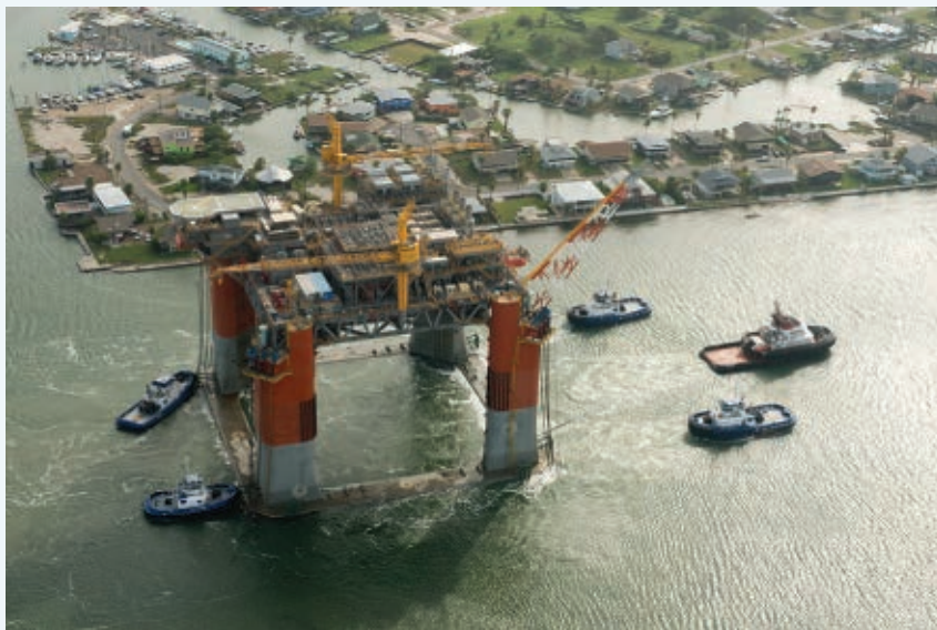
◀ Delta House FPS headed for service in Gulf of Mexico.
