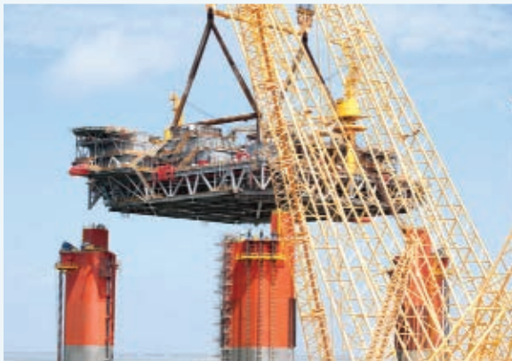
▲ Delta House being set on top of hull.
