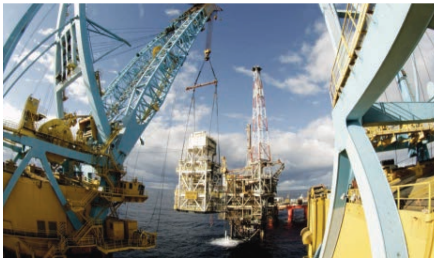
Module installation on the Andrew platform. (Photo courtesy BP)
