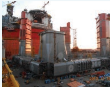
▲ Delta House hull in the shipyard.
