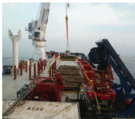
Mattress recovery operation offshore. (Photo courtesy Decom North Sea)
