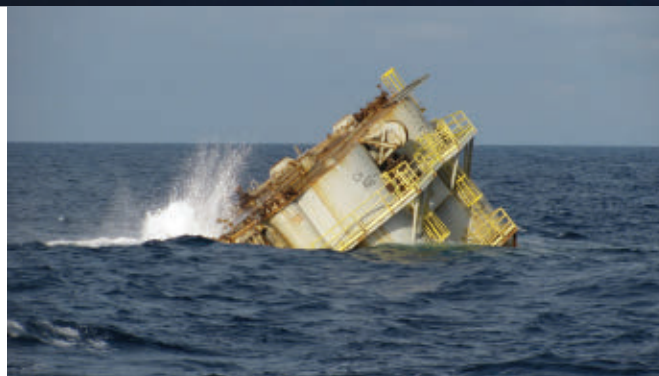
The Red Hawk spar was the first to be decommissioned in the Gulf of Mexico. (Photo courtesy InterMoor)
