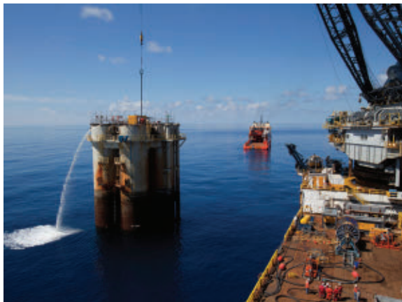
Deballasting following topsides removal. (Photo courtesy Anadarko)
