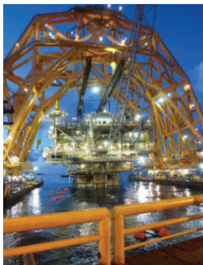
The VB 10,000 removes the Red Hawk cell spar's topsides. (Photo courtesy InterMoor)
