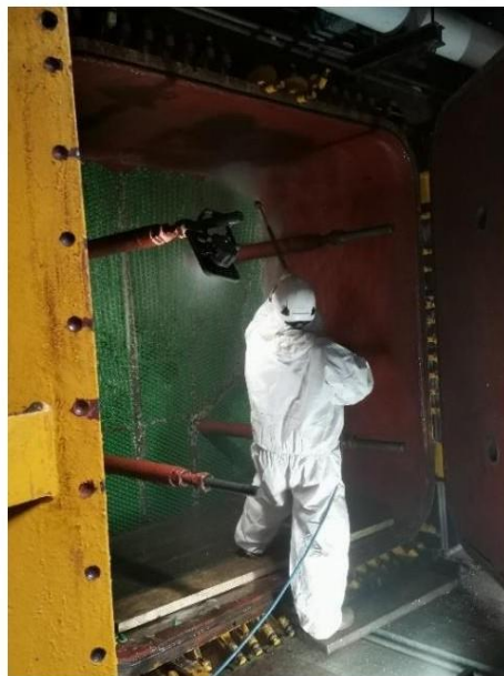
Fig. 2 - Installation Caps in PE Before of the sandblasting
