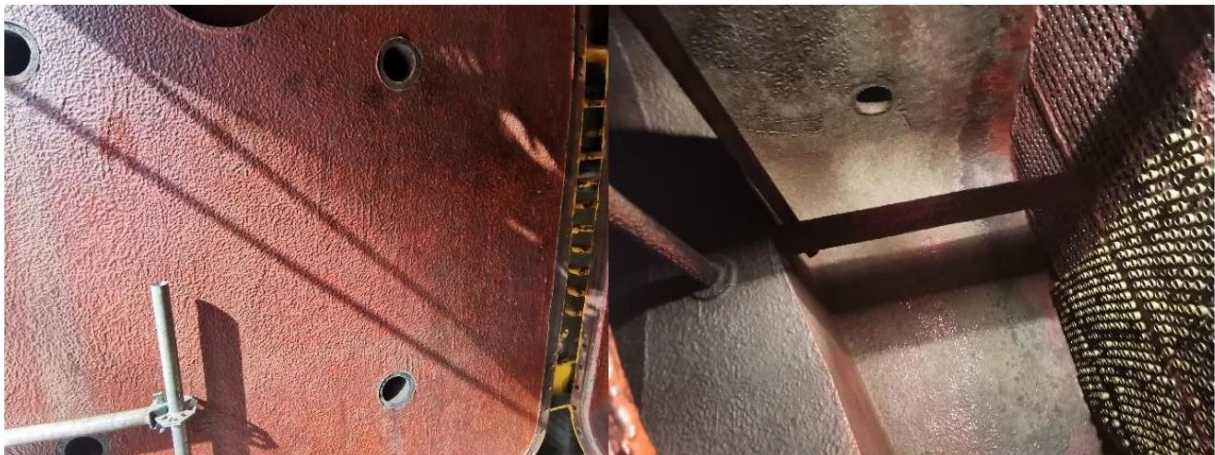
Fig. 1 - Image pre-works from plates tubes And speakers water; Evidence from a good level from storage of the speakers; the coating of the plates is state in great part for allow installation of the tubes.
