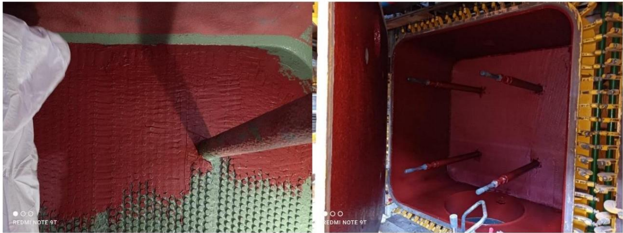
Fig. 6 - Application Phncote cladding system on plates tubes
