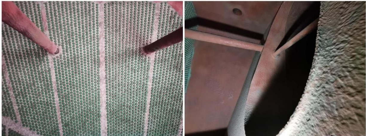
Fig. 4 - Preparation superficial plates tubes And speakers water
