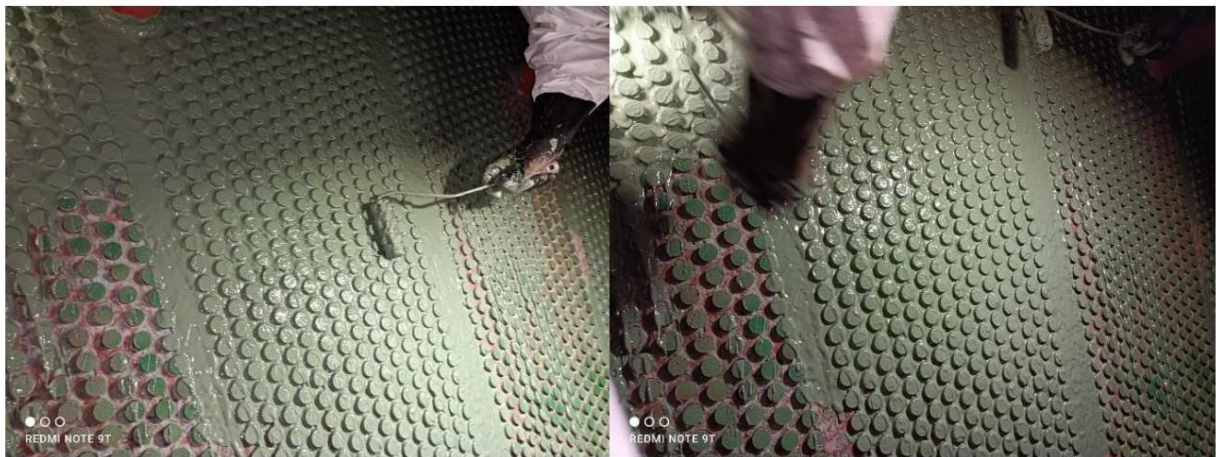
Fig. 5 - Application primer at plates tubes
