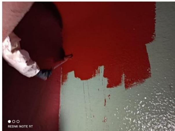
Fig. 8 - Application coating on water boxes
