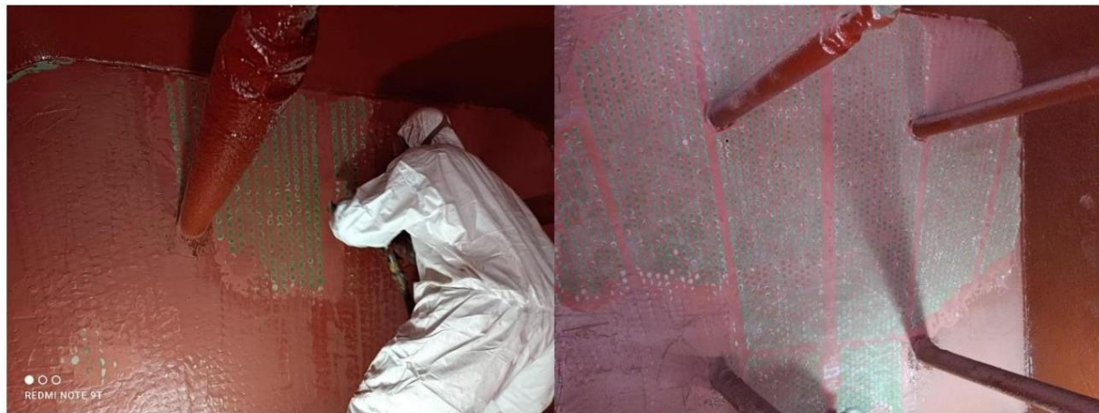
Fig. 7 - Sanding coating in Phoncote 2000 of the plates tubes
