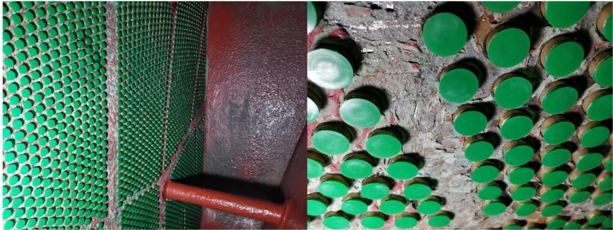
Fig. 2 - Installation Caps in PE Before of the sandblasting
