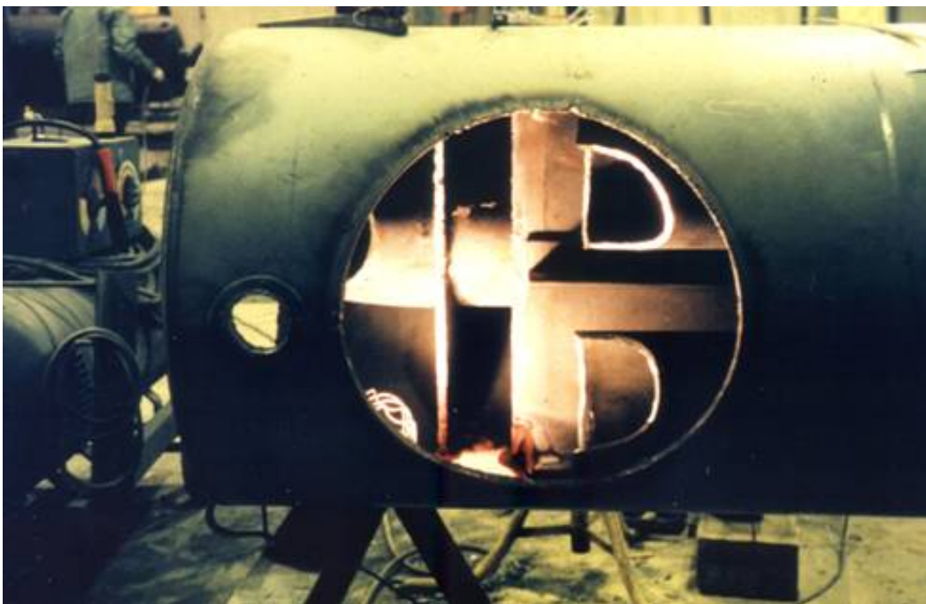
Figure 12 – Pulsation Bottle Internals Undergoing Repair
