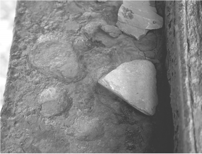
Fig. 2.12 Large holes created in a bridge structural steel by the presence of rocks. (Courtesy Kingston Technical Software.)
