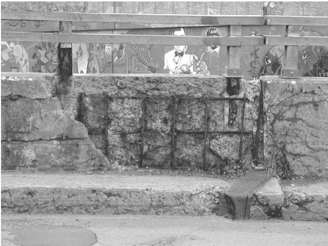
Fig. 1.9. Growth of the corrosion oxide products can lead to cracking and spalling of the concrete cover.
