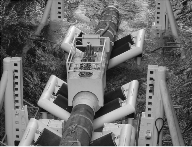
Fig. 4.9 A ring pair corrosion monitoring system being deployed at sea during the installation of a submerged pipeline. (Courtesy of Cormon Ltd.)
