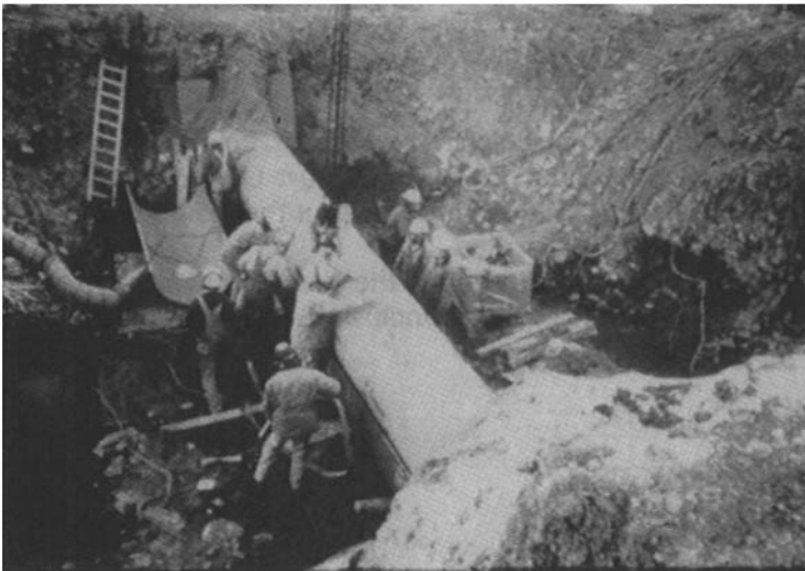
Fig.2. Corrosion inspection of the Trans-Alaska pipeline.
