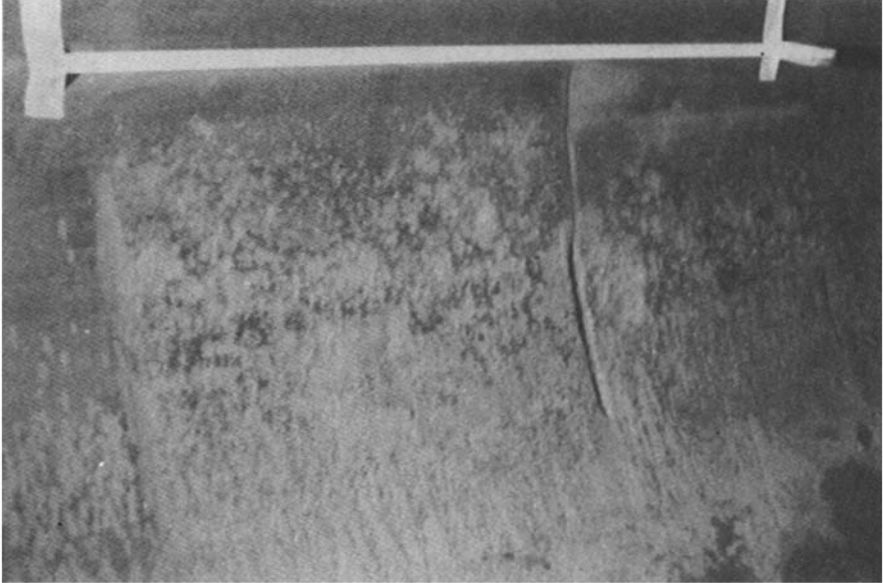
Photo 3. Internal natural corrosion sample on the girth weld in the test loop.
