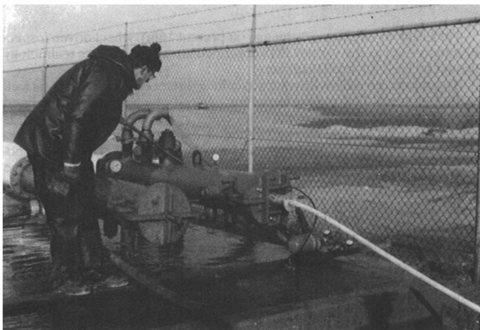
Fig.12. The stripper technique being used in the 10-in test loop.
