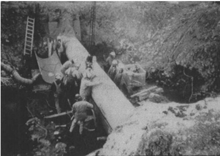
Fig.2. Corrosion inspection of the Trans-Alaska pipeline.
