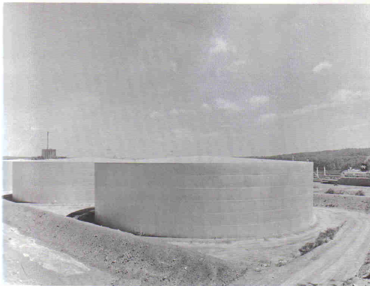
Figure 3-3. Cone roof tank. Courtesy of Chicago Bridge and Iron Co.
