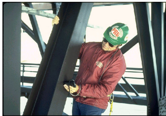
Inspection of Dry Film Thickness
