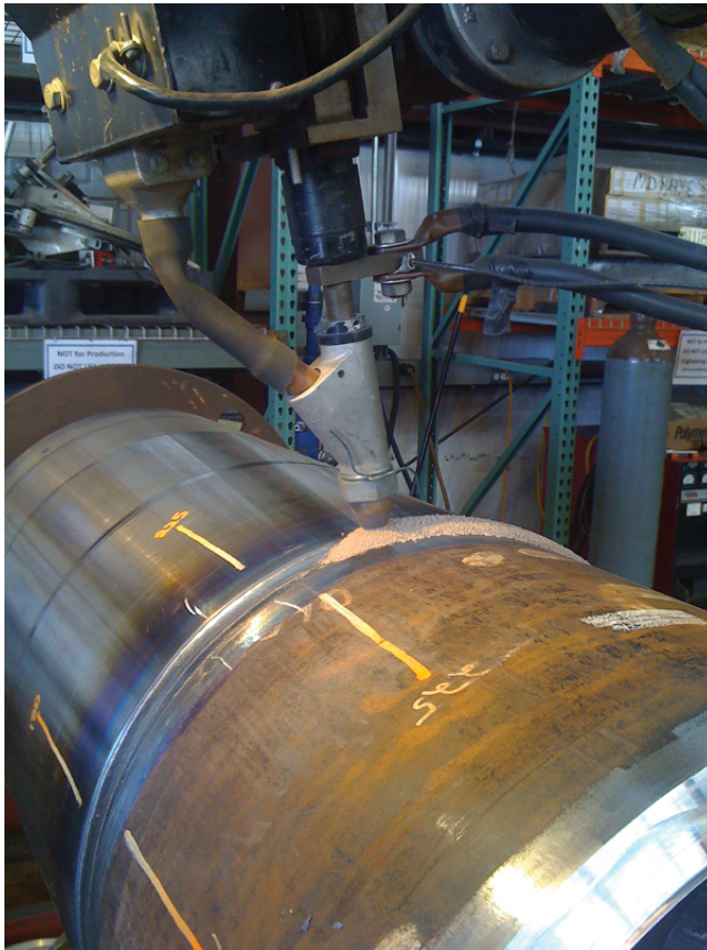
Figure 6.3.3 Shows the SAW of a pipe in a fabrication shop – note the arc and flux position as the pipe rotates.
