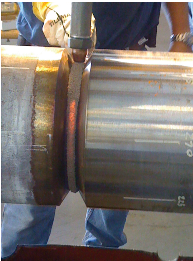
Figure 6.6.1 Showing SAW process in progress on a pipe weld.
