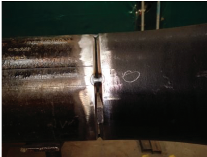
Figure 2.11.12 Weld tacks bridging two pieces of pipe.
