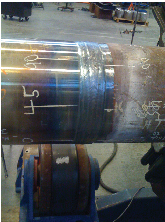
Figure 6.3.4 Shows the completed pipe weld.
