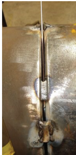
Figure 2.11.14 This picture shows both the bridge tack using external pieces of metal below, and just above that is the tack within the groove using welding.
