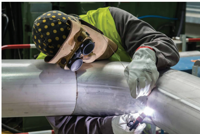
Figure 2.12.13 Pipe is assembled and prior to welding, the welder is tacking them with the GTAW process.
