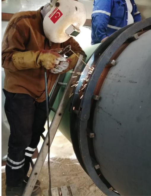
Figure 2.3 A SMAW welder welding on a pipeline project.
