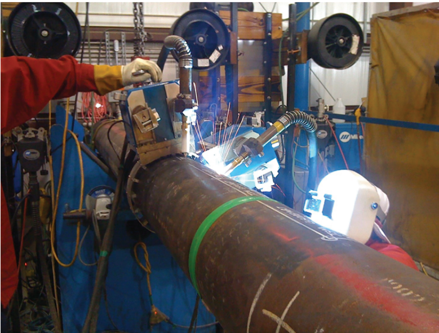
Figure 4.4.1 A GMAW operator welding on an offshore pipeline.
