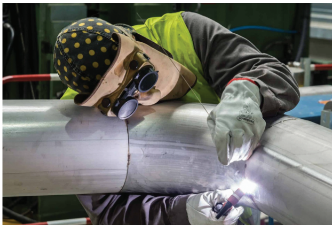
Figure 3.25.9.3.1 Welder is tacking a pipe prior to welding.
